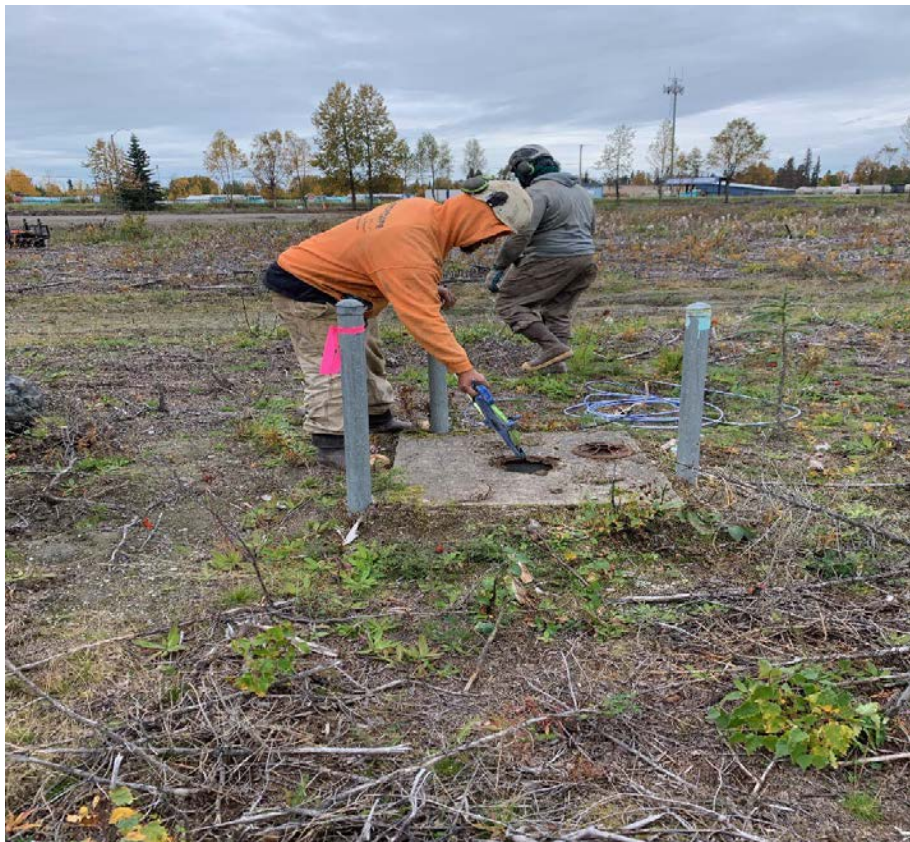
Photo #6: [Tank Farm, MW-30 Removal, Looking West, Photographer, Jacob Sweet]
