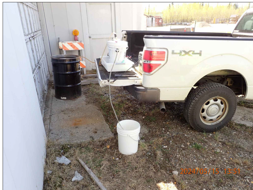
Photo 6: May 15, 2024. Looking south from the vicinity of the 4-Bay Building as the approximately 38 gallons of contaminated purge water generated from the six monitoring wells during sampling is processed and treated through a portable Granular Activated Carbon (GAC) system. The treated water was disposed of on Site by pouring to the ground surface a minimum of 100 feet away from drinking water wells or surface water.
