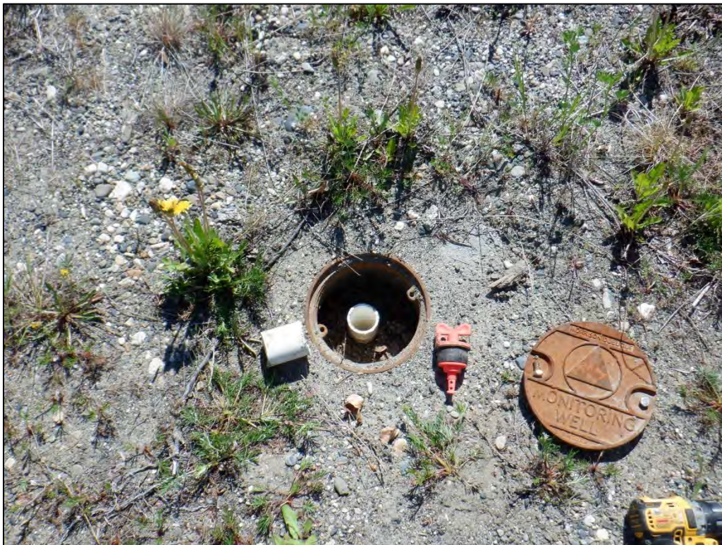
Photograph 4: 6/8/22. Trimmed approximately 2.75" of nearby MW-11 casing so that well cover fits.
