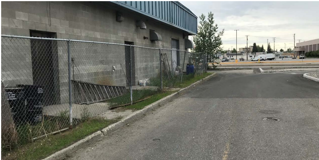
Exhibit 2-1: Various drums and containers at VIP Cleaners. Note the two 55-gallon PCE drums. The BMES upgradient monitoring well MW-1R is shown in the right foreground.
