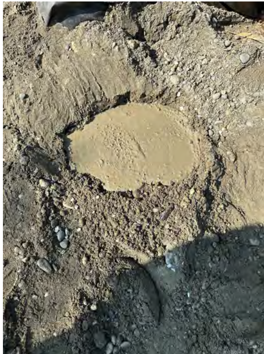
Photo 4: Cement cap placed to complete the backfilling of well M-3.
