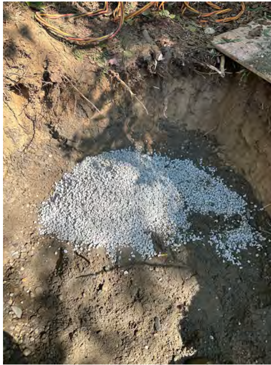
Photo 17: Bentonite chips placed on top of the cement cap at the Trailer Court Well.
