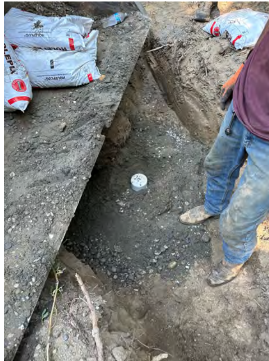
Photo 25: PVC cap glued on top of the well casing at well M-1.
