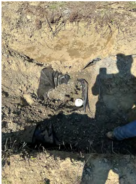
Photo 20: PVC cap glued on top of the well casing at well M-2.
