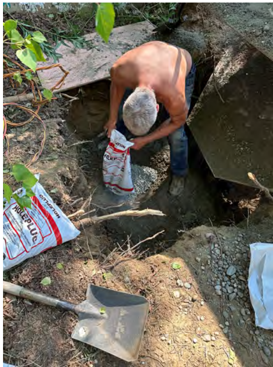
Photo 14: Backfill in progress at the Trailer Court Well.
