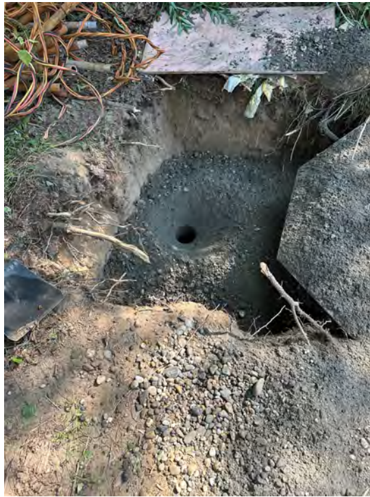
Photo 13: Backfill in progress at the Trailer Court Well.
