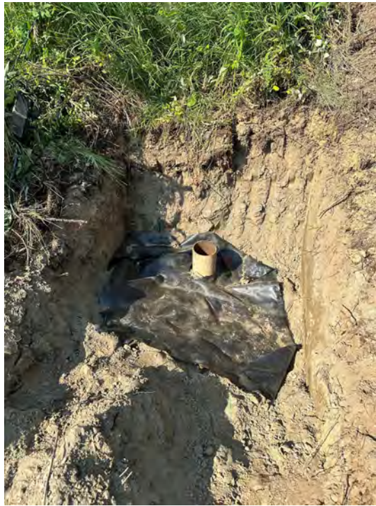
Photo 7: Excavation around the Pod Well in preparation for backfill.
