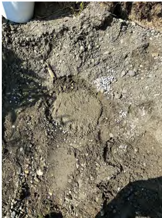
Photo 10: Cement cap placed to complete the backfilling of the Pod Well.
