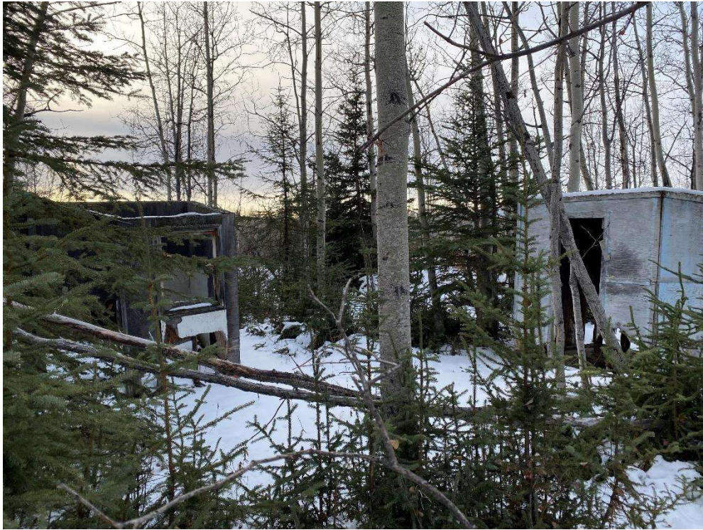
Photo 13: Test Grids 3-7/CRREL Areas F, G, and H. Abandoned shacks in the northern area of the site.
