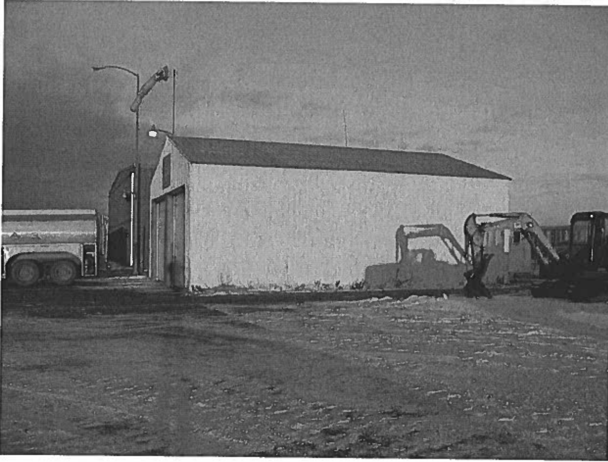
Photo: 2 Time: 0959 Date: 10/12/2007 Direction: West Subject: Crowley Hangar.
