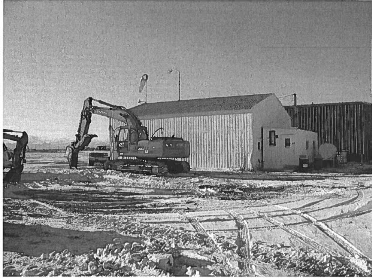
Photo: 13 Time: 1437 Date: 10/12/2007 Direction: Southwest Subject: Excavating at Test Pit 4 (T4).
