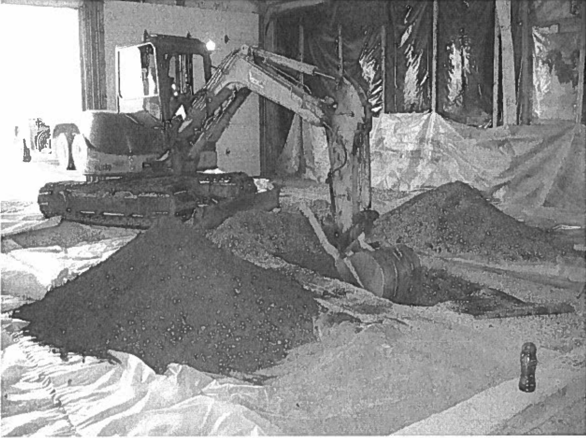
Photo: 9 Time: 1052 Date: 10/12/2007 Direction: South Subject: Excavating Test Pit 1 (T1).
