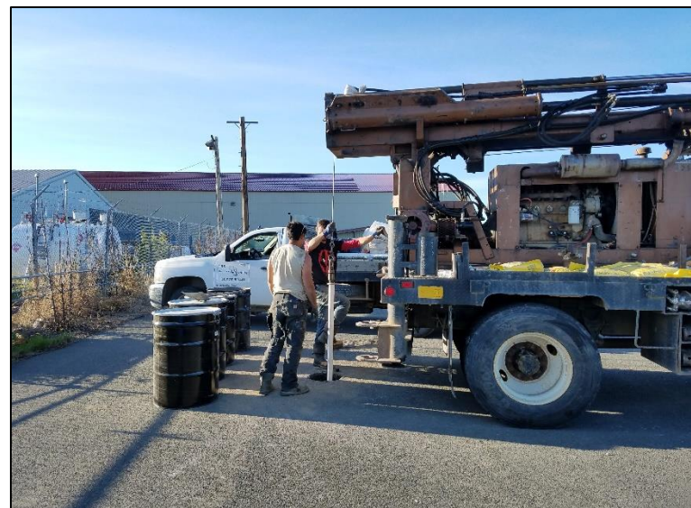
Decommissioning RSE-1 following sampling.
