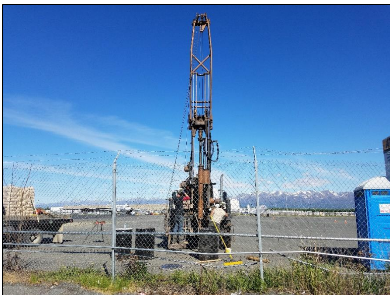
Drill rig setting up at RSE-1, facing east.
