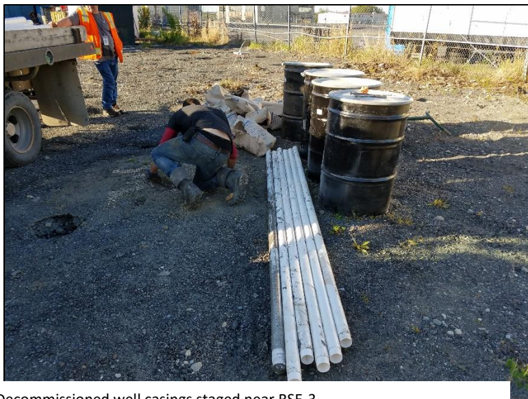
Decommissioned well casings staged near RSE-3.
