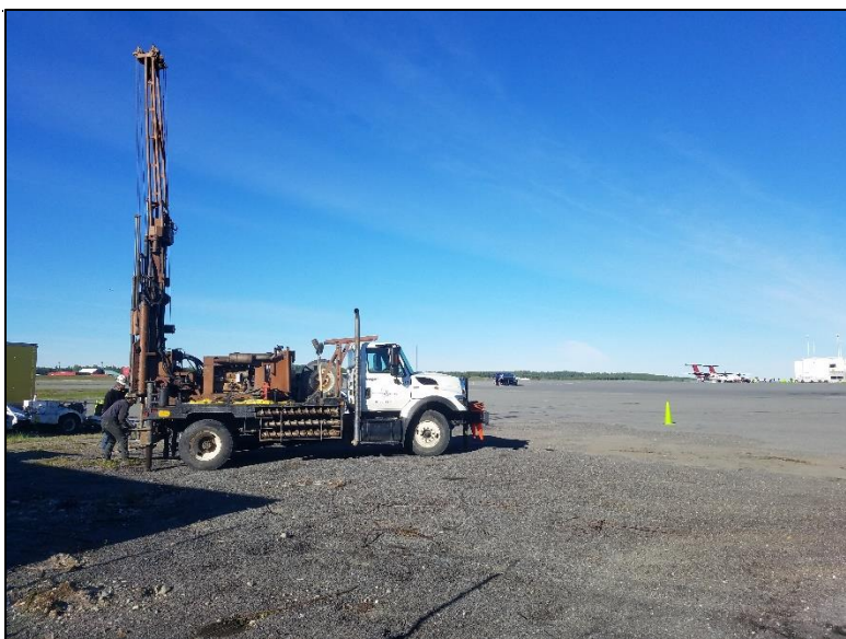
Mobilizing drill rig to RSE-3.
