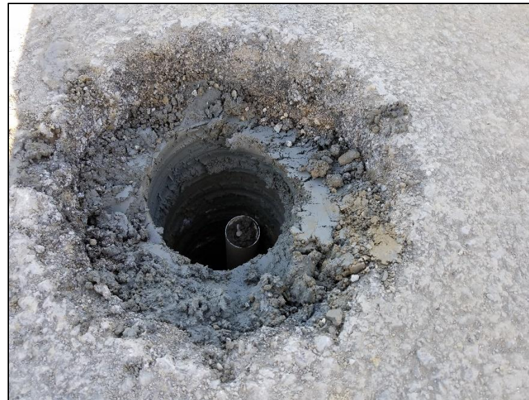
RSE-1 recessed temporary monitoring well.
