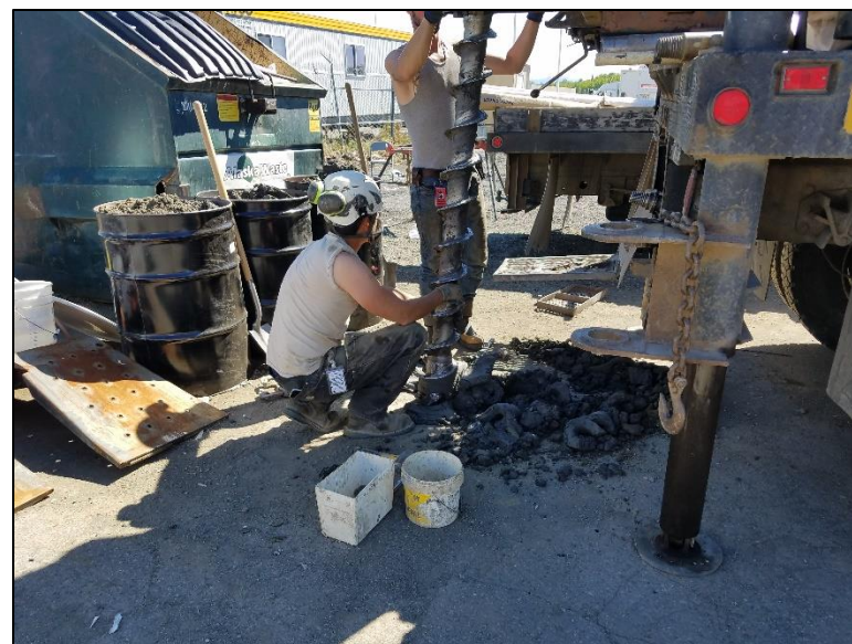
Installation of temporary monitoring well at RSE-2.
