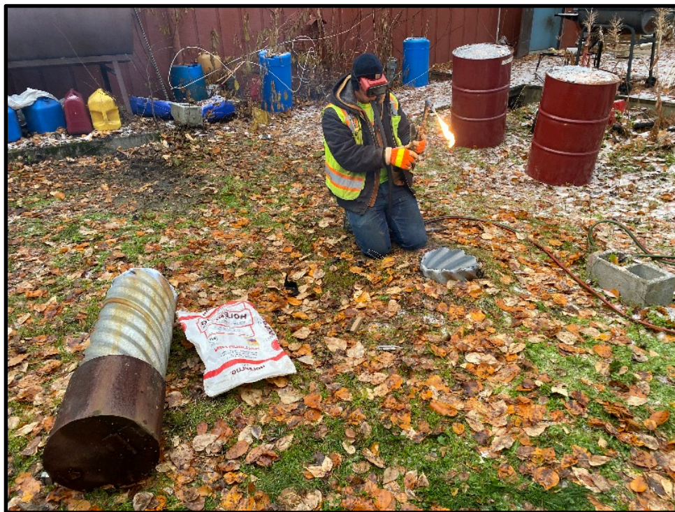
Photo 6: Cut the culvert recovery 2' below ground level with an acetylene torch
