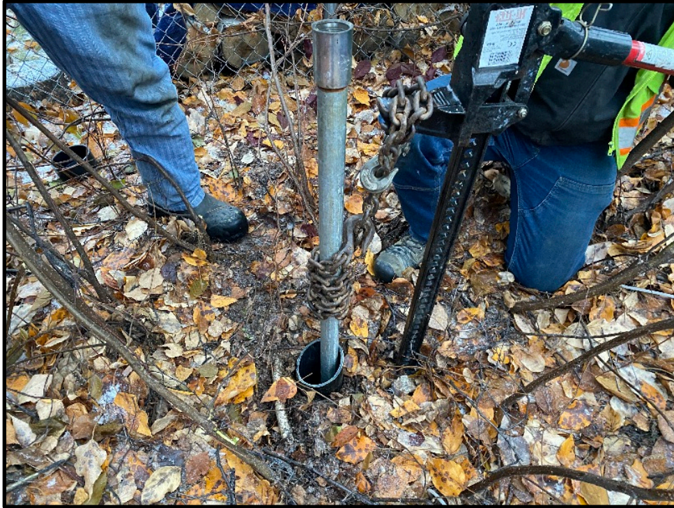
Photo 1: (MW3) pulling the galvanized well pipe out of existing ABS piping
