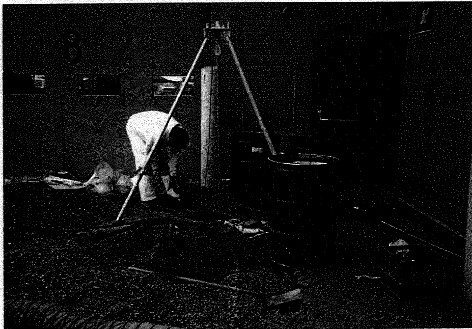
Photo 4: Rowcon personnel entered and cleaned the UST. 150 gallons of used oil were removed.
