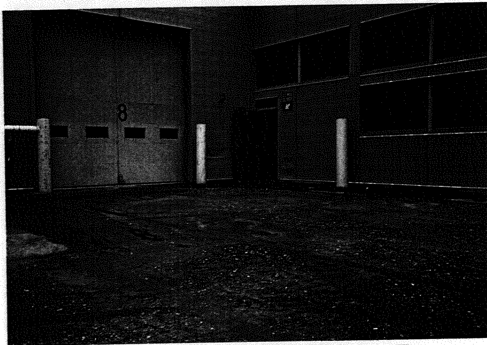
Photo 6: The tank manhole and overflow pipe were cut down and sealed, as were underground pipes leading to building. Site was backfilled and restored.
