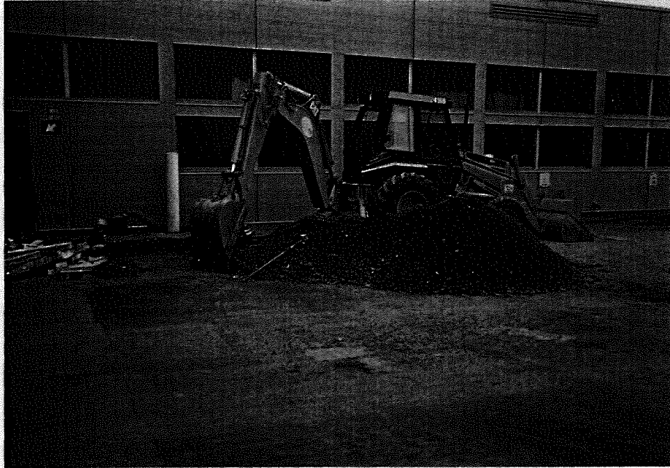
Photo 3: Soil stockpile and view of one-story maintenance complex. Excavation was limited to safe distance from the building (on the west side and south end).
