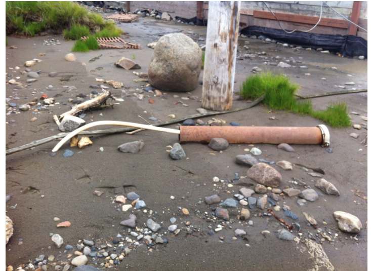
Photo 10. PZ-2 Before Replacement in 2013
