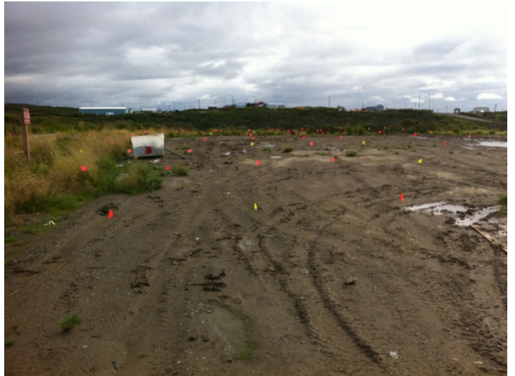
Photo 4. Establishing Grid for MI Sampling of Land-Farm
