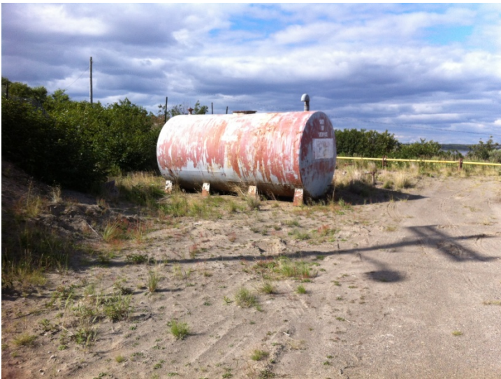
Photo 15. Out-of-Service 3,000-Gallon Aboveground Storage Tank Near Tank Farm
