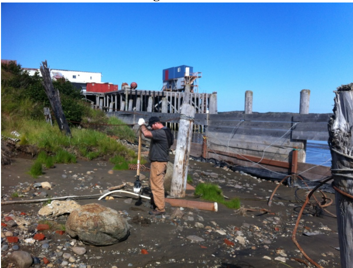
Photo 11. Replacing PZ2, Inter-Tidal Area of Beach
