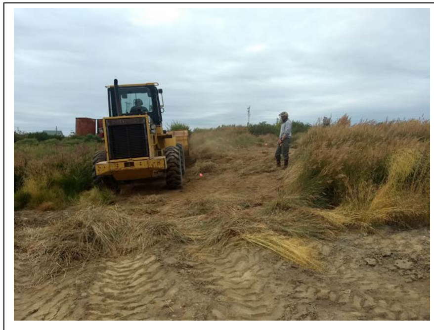
Photo 2: Looking west while clearing vegetation from the surface of Landfarm Area 1 (Decision Unit DU1). (August 12, 2019)
