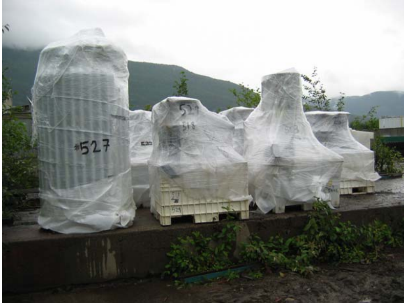
Photo 20: Transformers 518, 519, 527, 7525100, 529, 516, 520 and expansion tank for 503 drained and temporarily stored for shipment
