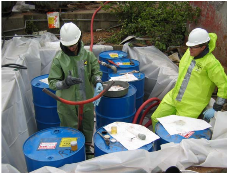
Photo 12: Transformer draining and rinsing using lined containment basin from former dip tank
