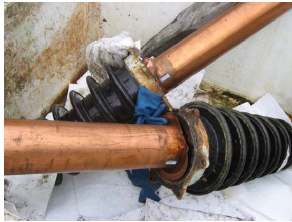
Photo 11: Two of 6 insulators overpacked for disposal
