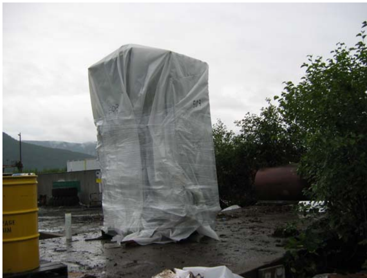
Photo 19: Transformer 503 drained and temporarily stored for shipment
