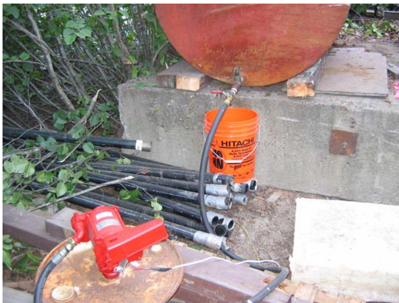
Photo 12: Transformer draining and rinsing using lined containment basin from former dip tank
