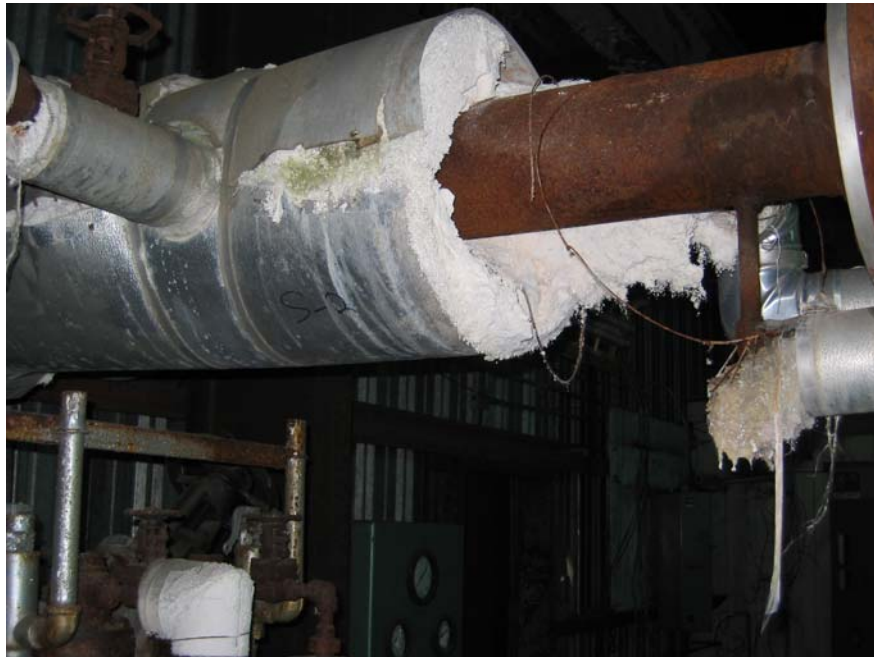
Photo 2: S-2 Pipe Insulation from 2 nd Floor; Result Non-ACM
