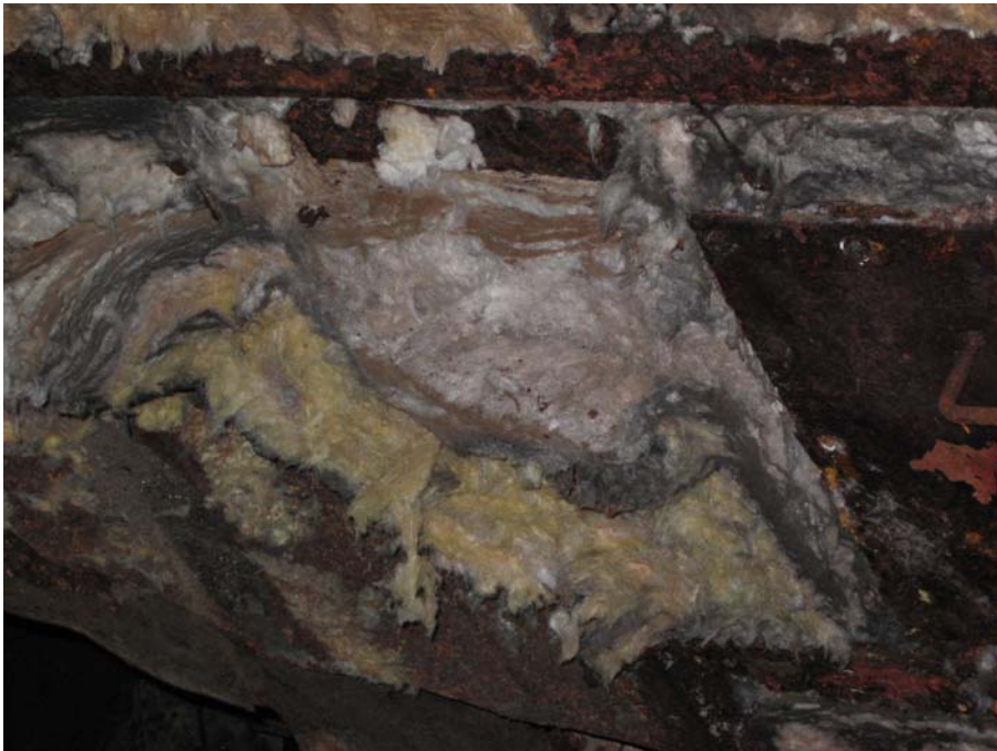
Photo 6: S-8 Insulation under Furnace Area; Result Non-ACM
