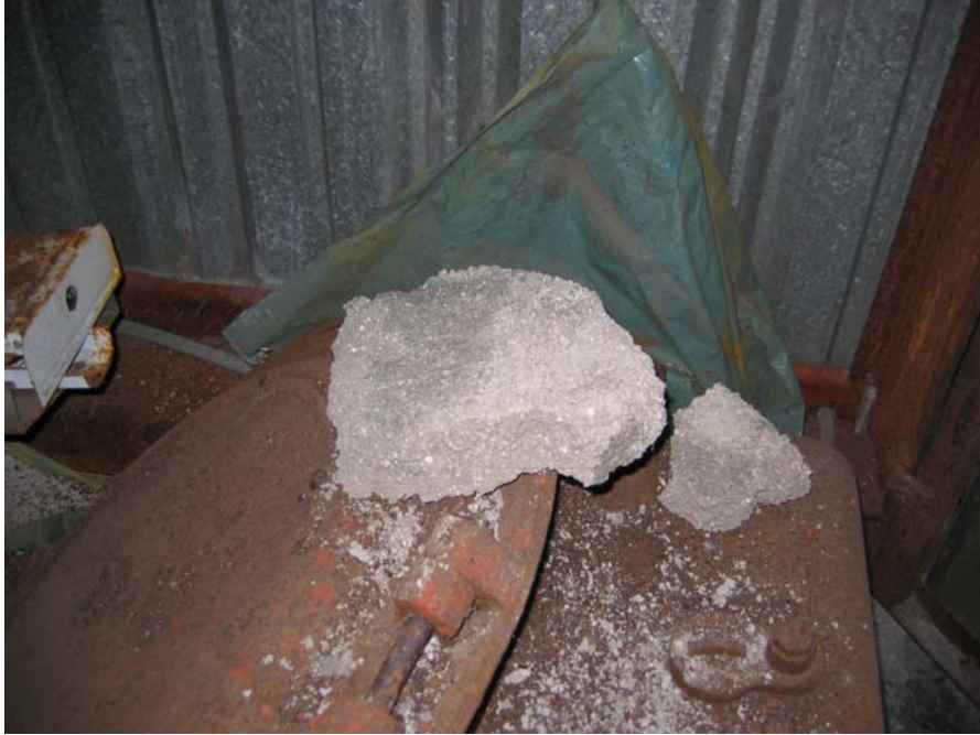
Photo 5: S-7 Granular Insulation in Basement; Result Non-ACM
