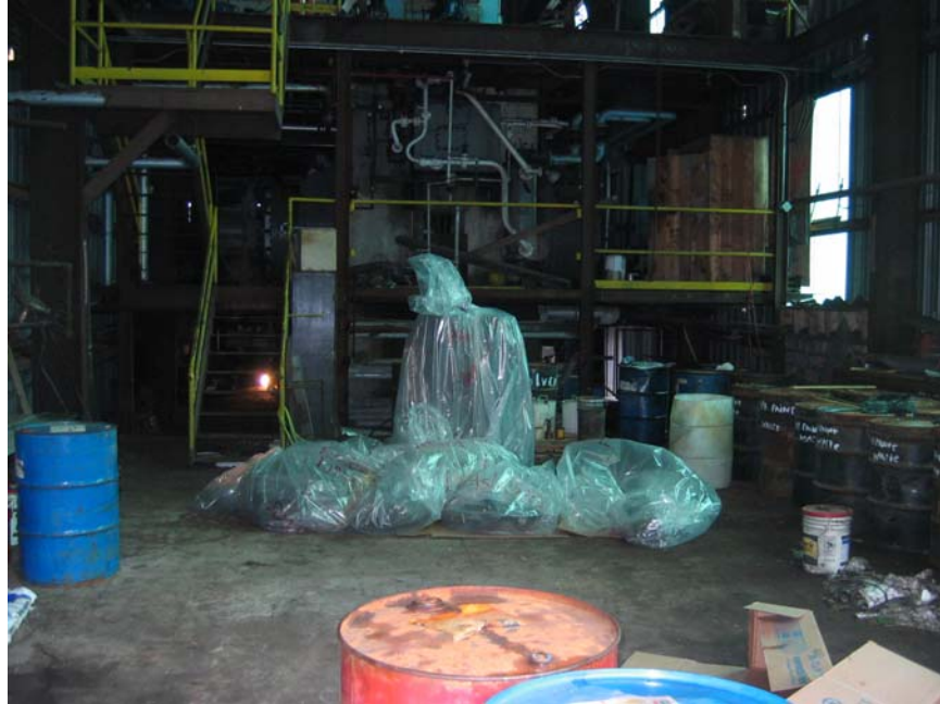
Photo 13: Asbestos Materials Double Bagged for Removal to Approved Facility
