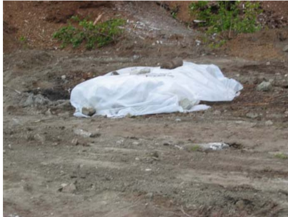
Photo #11 Asbestos concrete board
