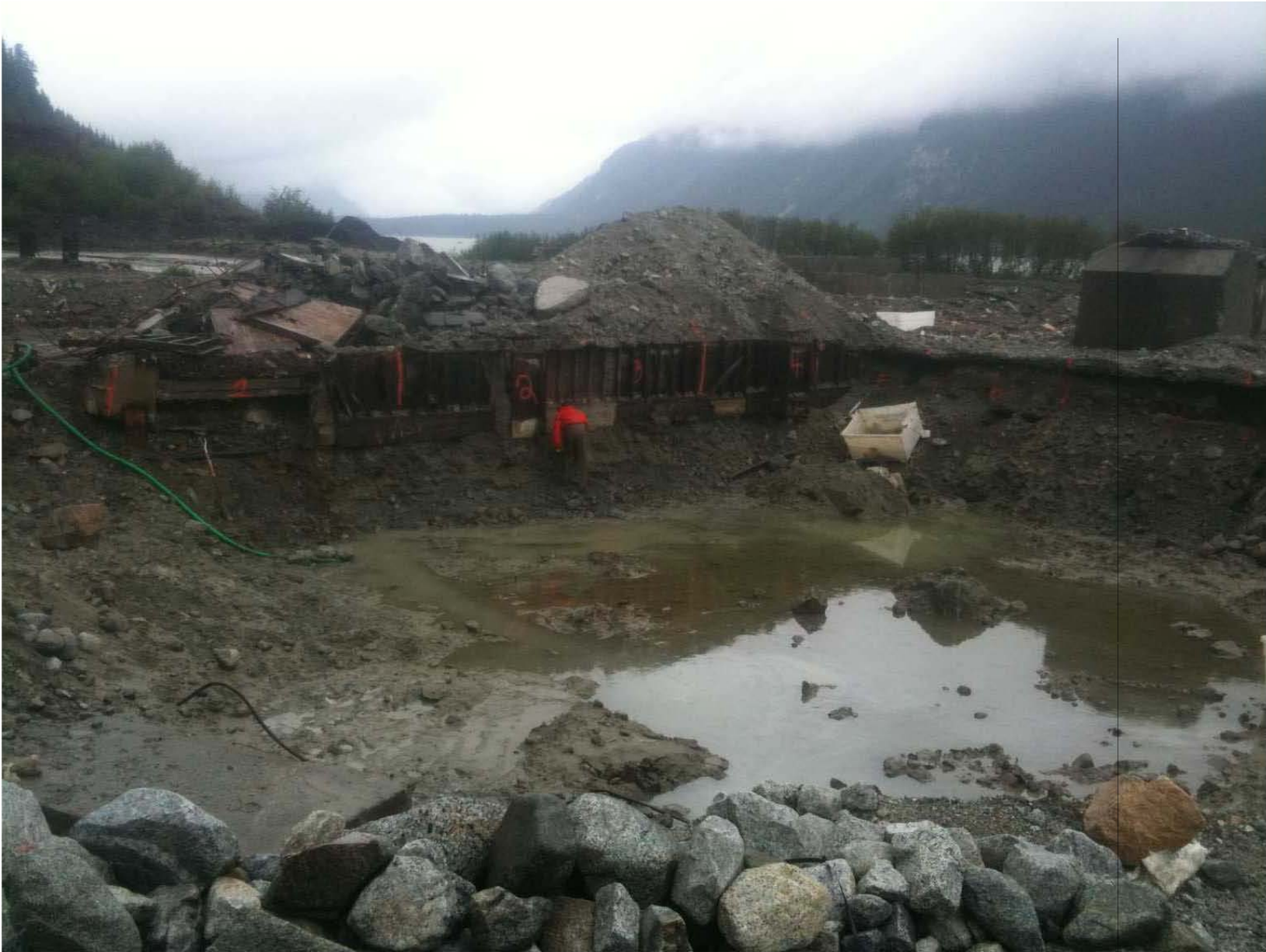
Photo 1: Extent of powerhouse shop excavation
