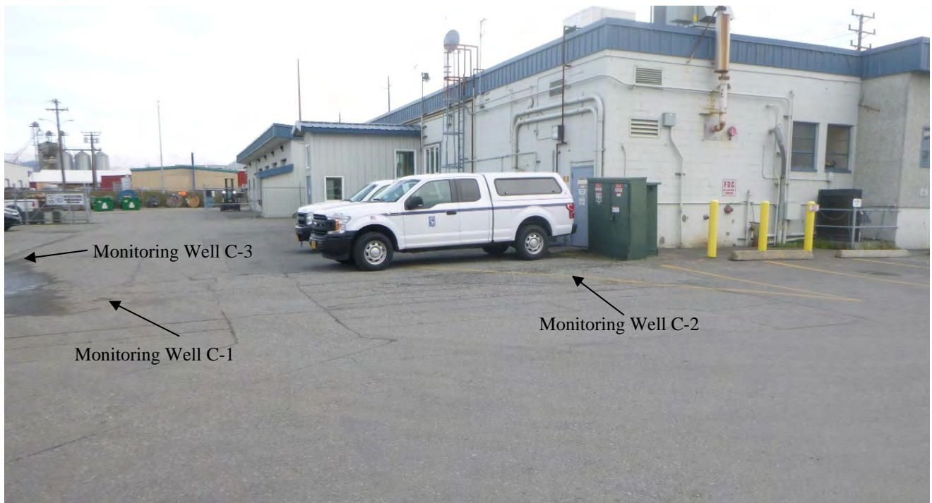
Photo 6: Operations and Dispatch Center from the west. Approximate well locations are shown. The trucks are parked over the approximate source area (PCB impacted soils below asphalt pavement, see Figure 2). (10/16/20)
