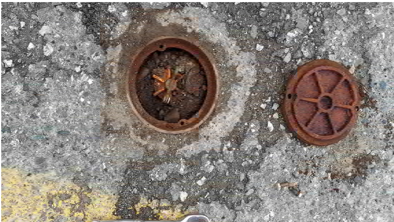
Photo 2: Well C-2 on July 2, 2021 prior to maintenance and groundwater monitoring. On July 7, 2021 the well was cut down by 2 inches and the excess bentonite was removed. (7/2/2021)
