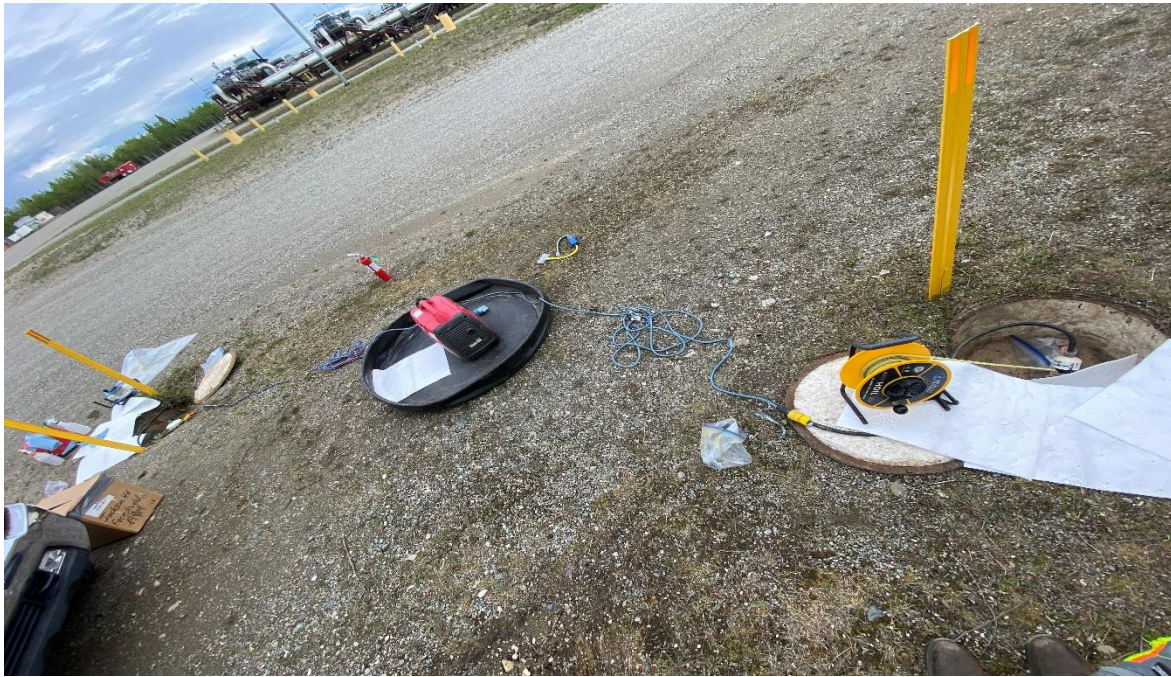
Photo 2: Product recovery equipment set up at MW-5 (June 27, 2024)
