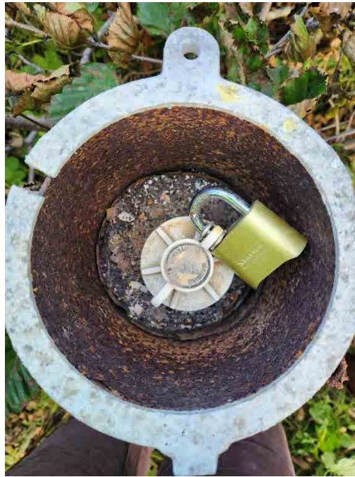
Photo ID: 1. Well ST005-MW3 locked. Well monument was not locked from outside and well was not labeled.
