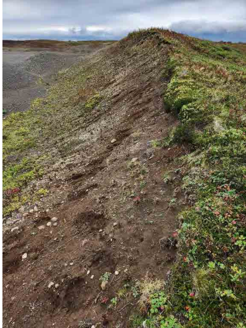
Photo ID: 45. View east. Possible unstable slope next to gravel borrow pit on north side of LF002.
