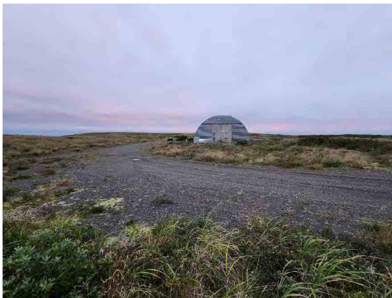
Photo ID: 59. View northwest. Entrance to site OT001 and access road in good condition.
