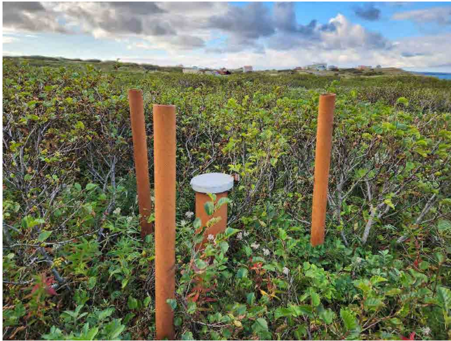
Photo ID: 11. View west. Well ST005-MW6 not properly locked and not labeled.
