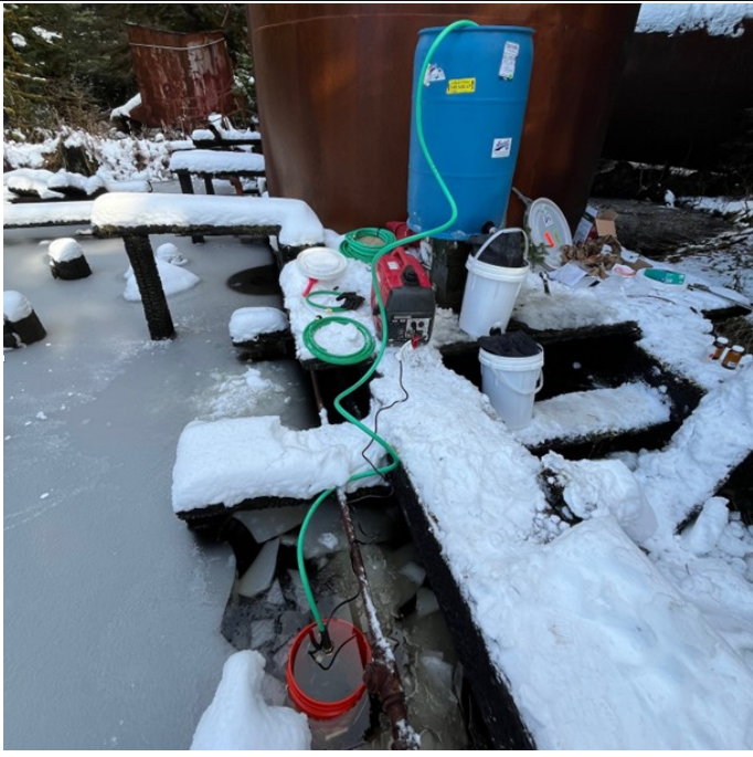
Photo showing the propped treatment system setup within the facility's secondary containment.
