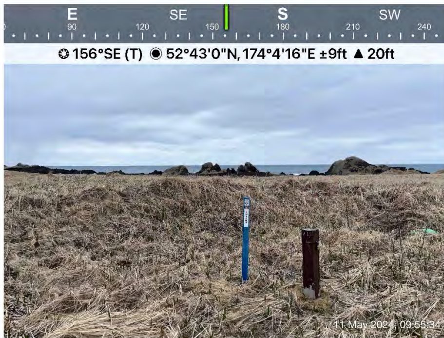
Photograph 14: LF024 groundwater monitoring well SW10W3.
