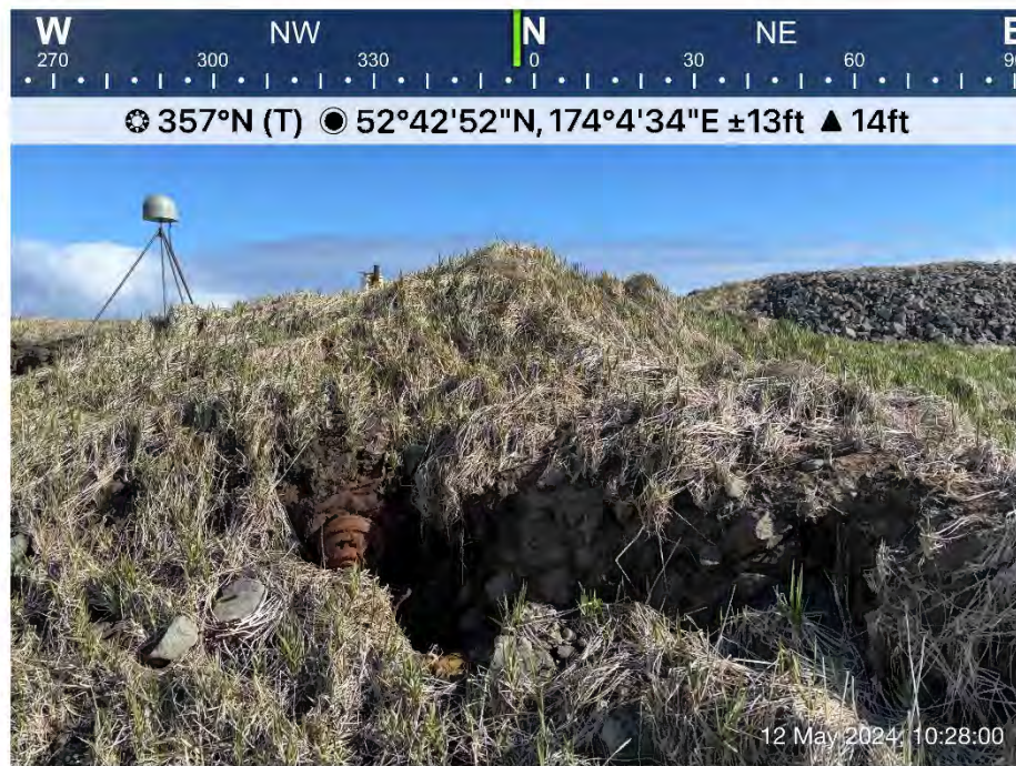
Photograph 36: LF026 exposed landfill debris in cover slough below the CORS station.
