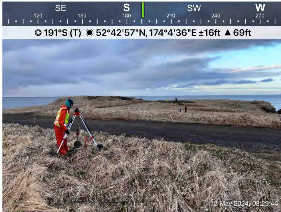
Photograph 37: Landfill survey control point location across from LF026.
