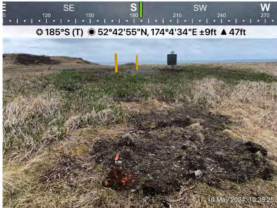
Photograph 35: Disturbed landfill cover with exposed debris from recent electrical upgrades.
