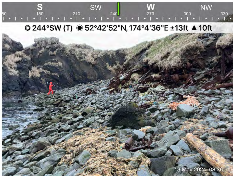
Photograph 32: GPS survey of LF026 southeastern boundary exposed landfill debris in the middle to high intertidal zones.
