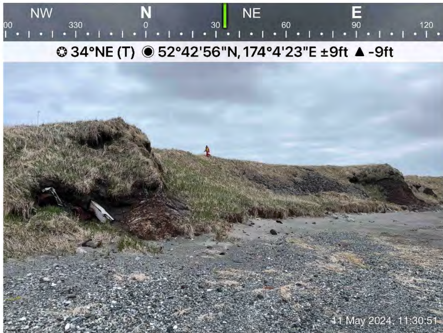
Photograph 20: Buried metal and wood debris in the eastern beach bluff.
