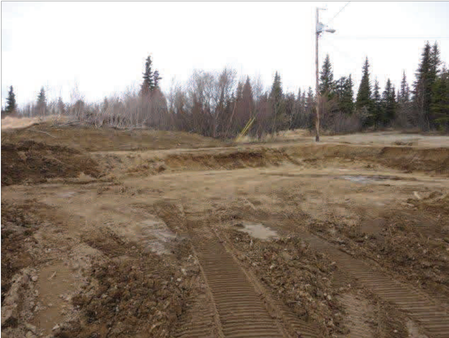
Former Stockpile Area
