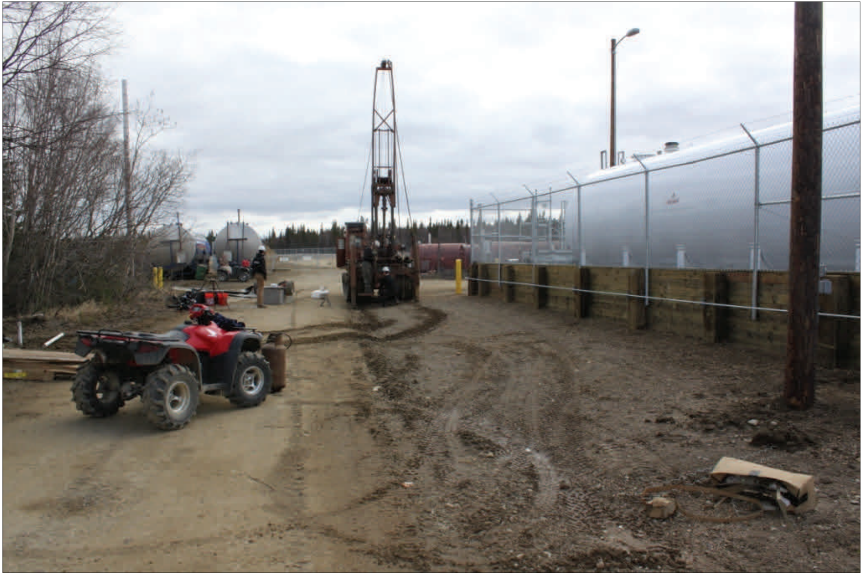
Bore Hole #2—SE Corner of New Tank Farm
