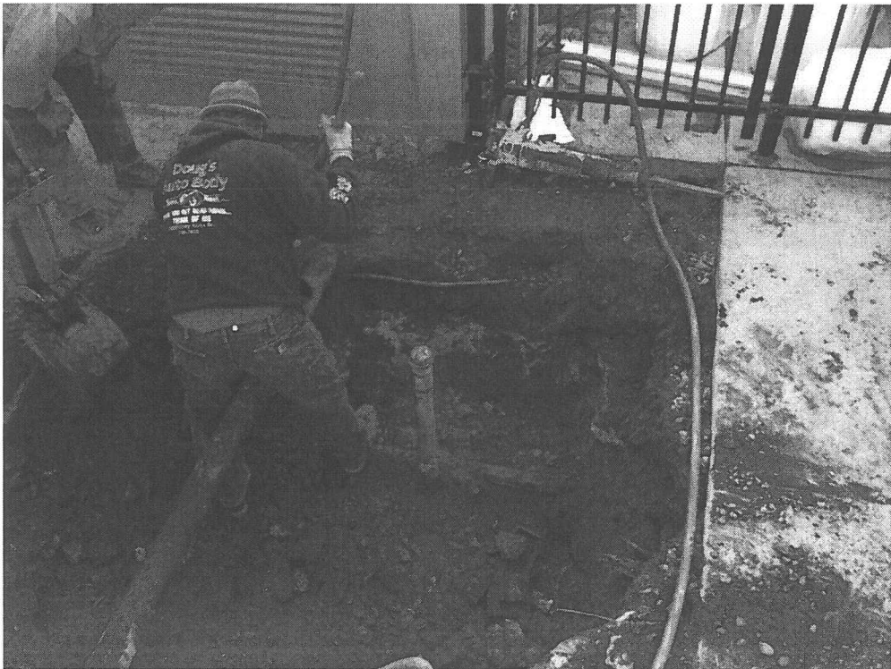
Photo 4: The second concrete slab is seen approximately two feet below the existing slab
