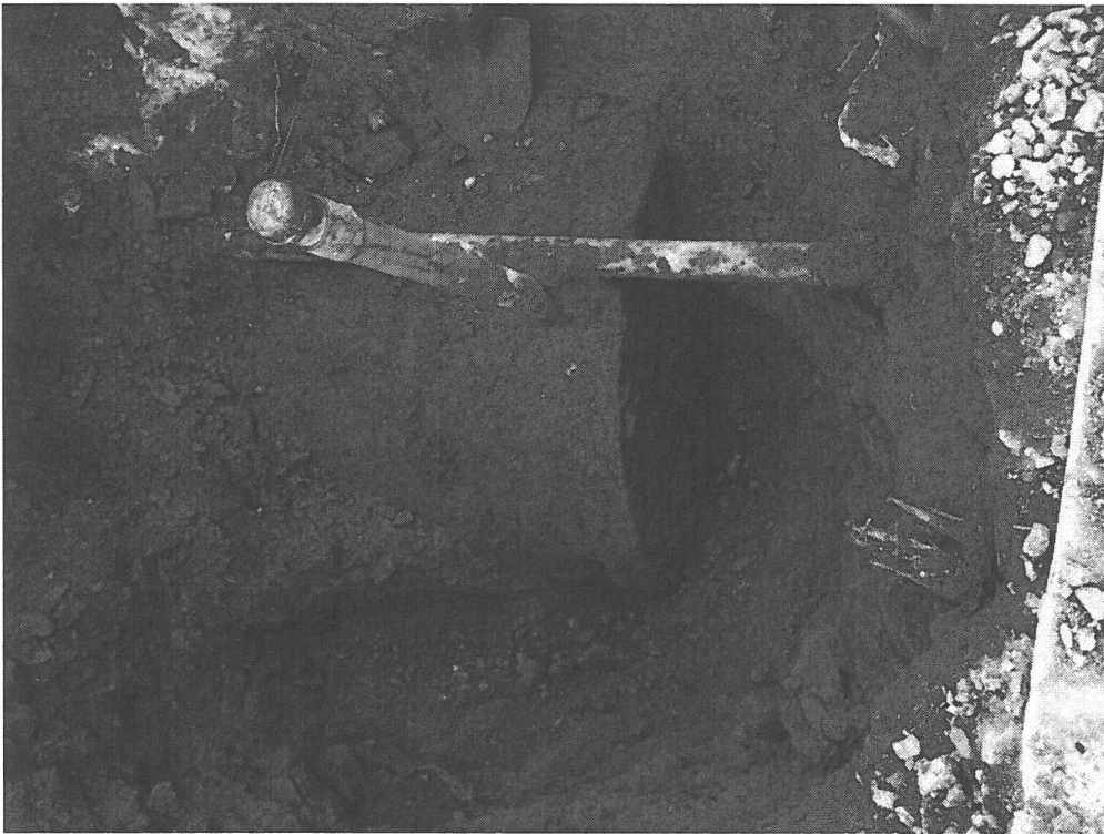
Photo 3: The 675 gallon tank starts to get exposed. Note other utility piping beside fill pipe.
