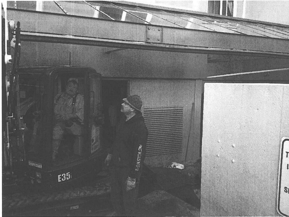
Photo 5: Low clearance for equipment posed an additional challenge for site work.
