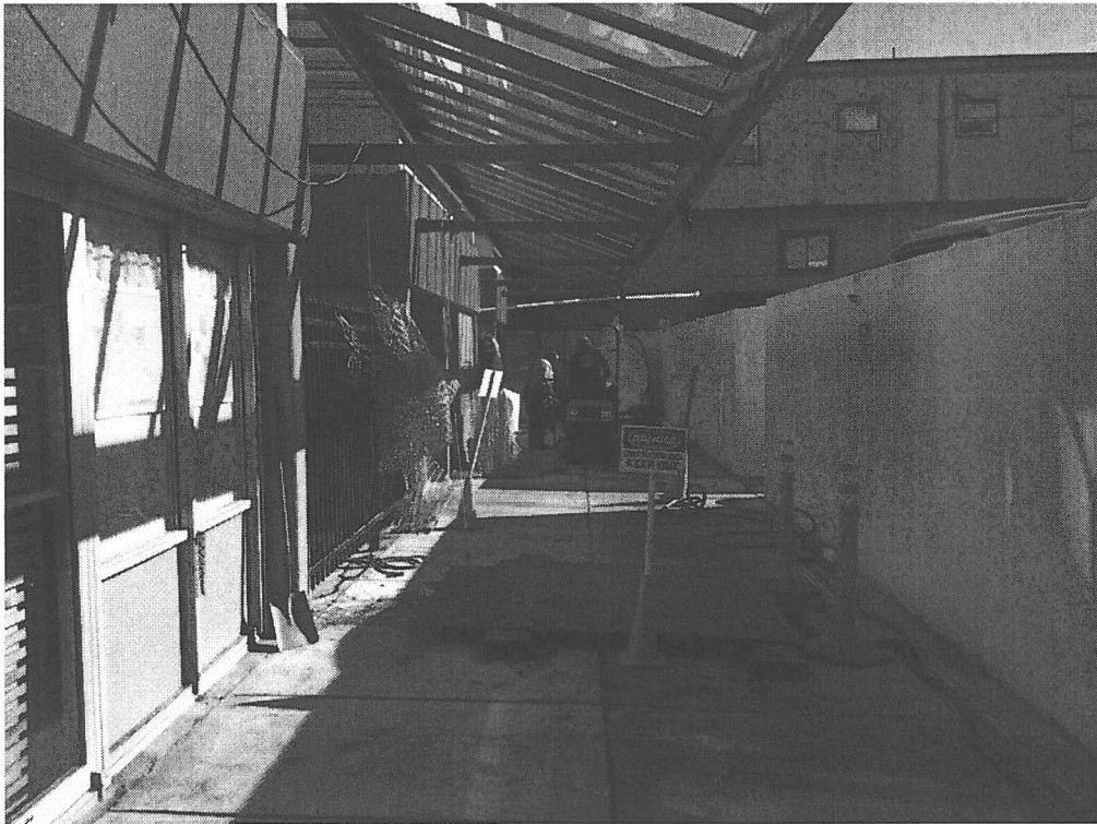
Photo 1: View of the tank area looking generally south. The awning and parking lot proximity limited site access to larger equipment.
