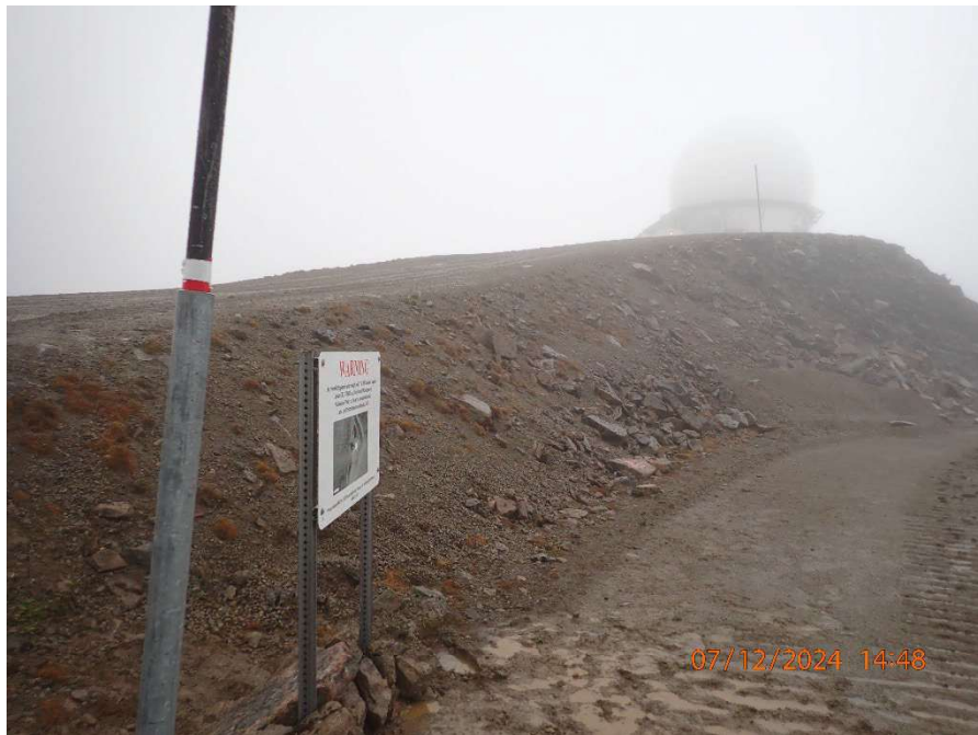
View north. New location of LUC sign removed from north side of SS016 building showing proximity to access road and building.
