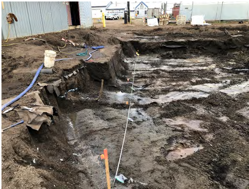
Photograph 1: First row of headspace samples within the contaminated soil excavation.
