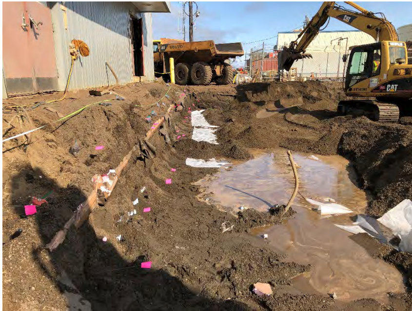
Photograph 4: Field-screening and sampling the western extent sidewall.
