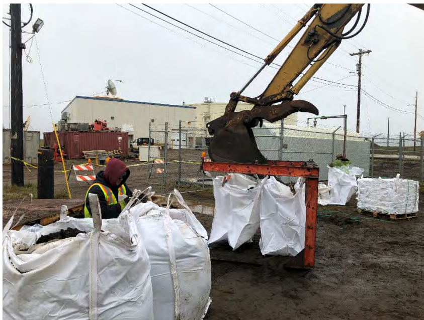
Photograph 2: Excavating potentially contaminated soil into supersacks.
