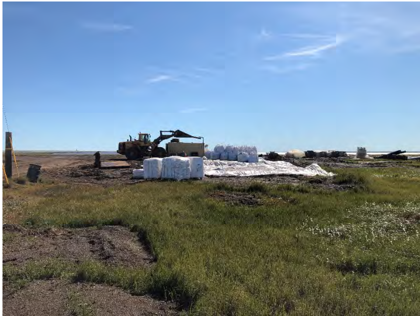
Photograph 4: Supersacks staked at the staging area located at the old airport.
