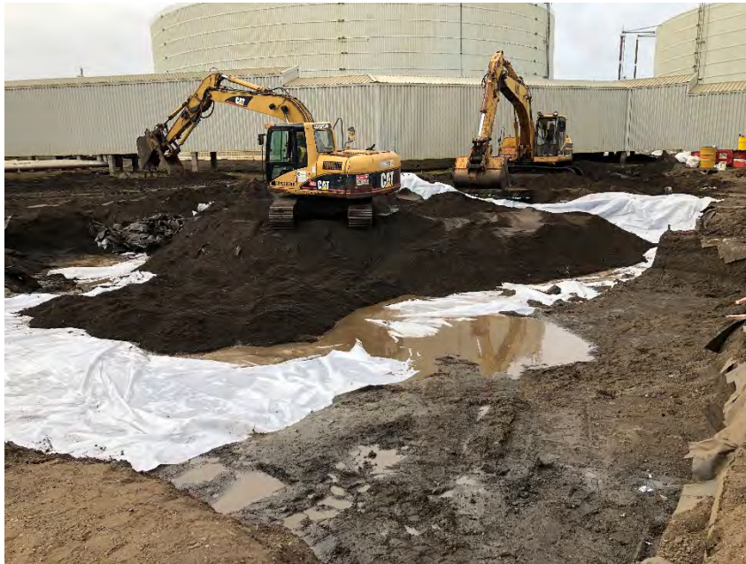
Photograph 2: Deploying visqueen and gravel over a finished portion of the excavation.
