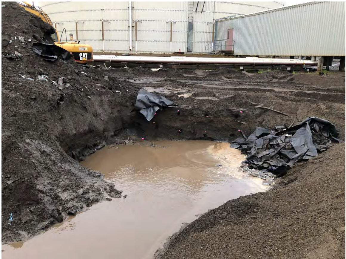
Photograph 1: Field-screening and sampling the northeastern sidewall of the expansion area footprint.
