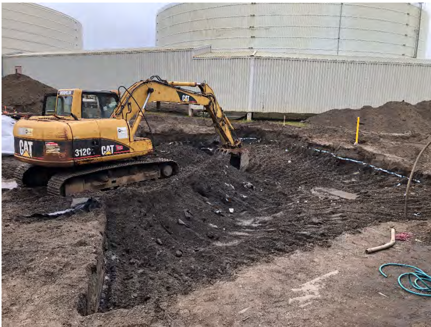
Photograph 2: Contaminated soil excavation as of 8/5, facing southeast.
