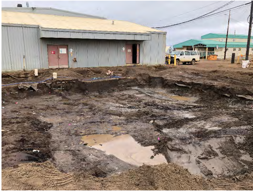
Photograph 2: Base of excavation analytical sample locations marked with pink pin flags.
