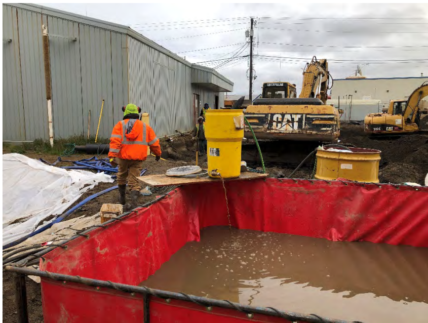
Photograph 5: Treating the water contained in the temporary holding pond with GAC.
