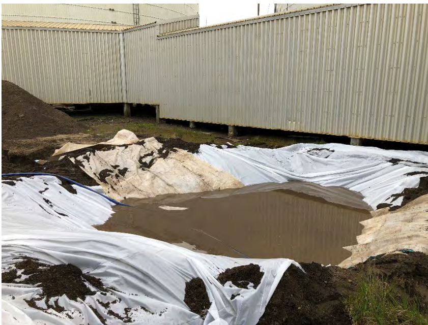
Photograph 2: Temporary containment pond constructed near the southeast corner of the WTP.
