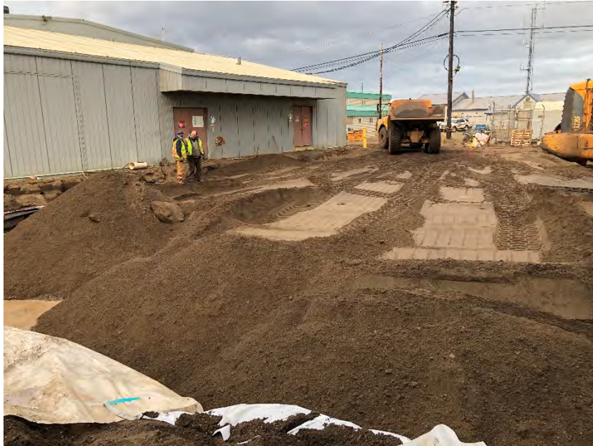
Photograph 4: Backfilling the southern end of the expansion area footprint.
