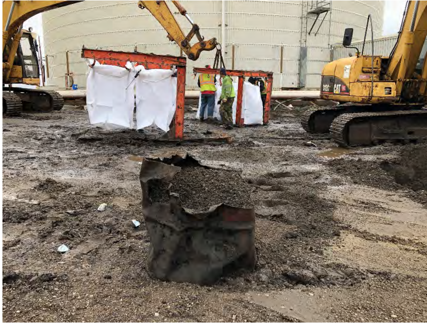
Photograph 1: A partial drum exposed while excavating the northeast corner. No discernible odor or trace of fluid observed.
