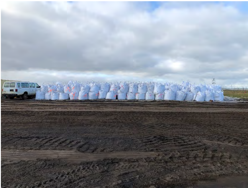
Photograph 3: The supersack staging area at the old airport as of 8/11/21.
