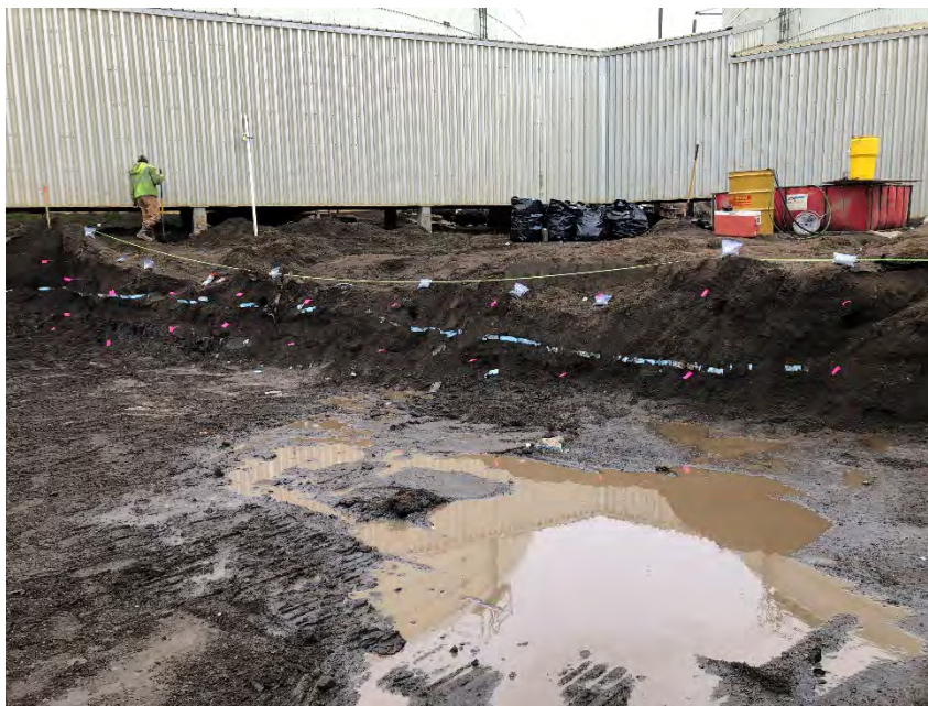
Photograph 1: Field-screening and sampling the southern sidewall of the expansion area footprint.
