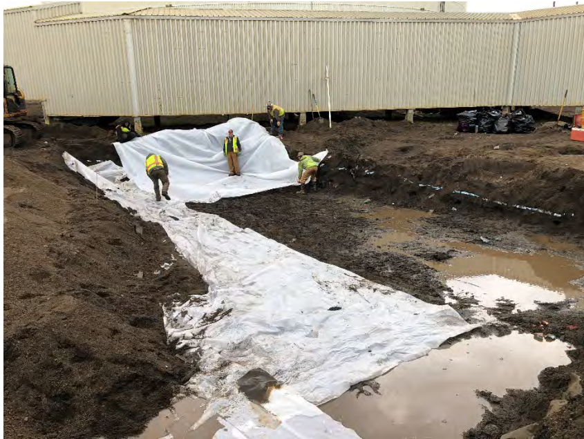
Photograph 3: Deploying visqueen over the southern end of the expansion area footprint.
