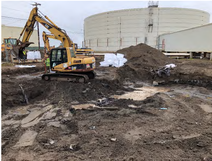
Photograph 1: Excavating and containerizing contaminated soil from below 2' bgs, facing east.
