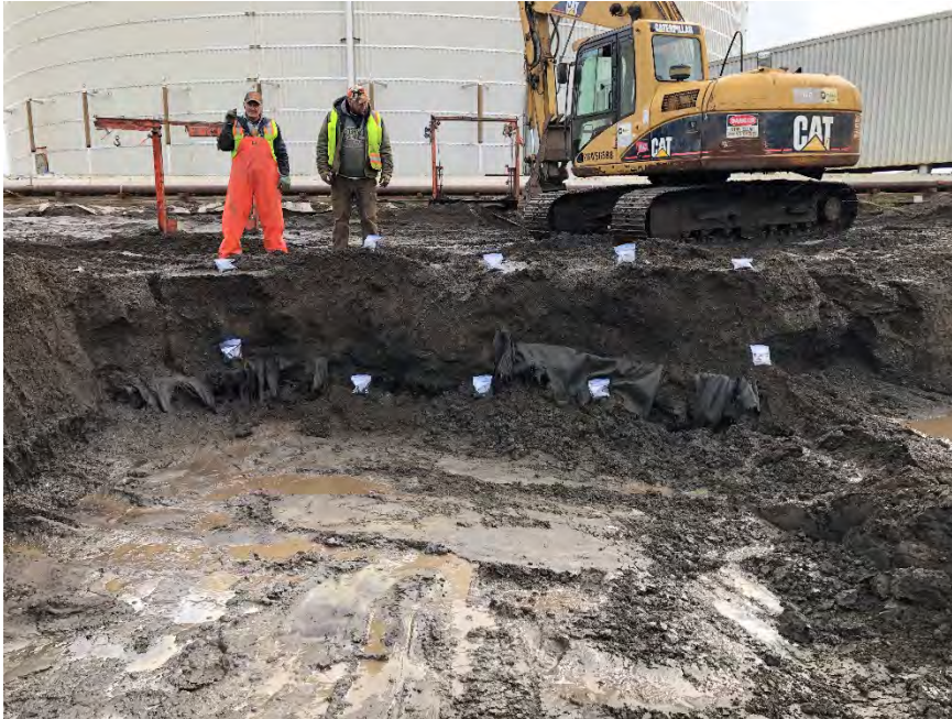
Photograph 3: Field-screening the remaining portions of the sidewalls at the northeast corner.
