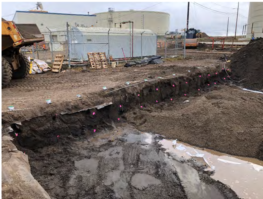
Photograph 3: Field-screening and sampling the accessible portion of the northern extent sidewall.
