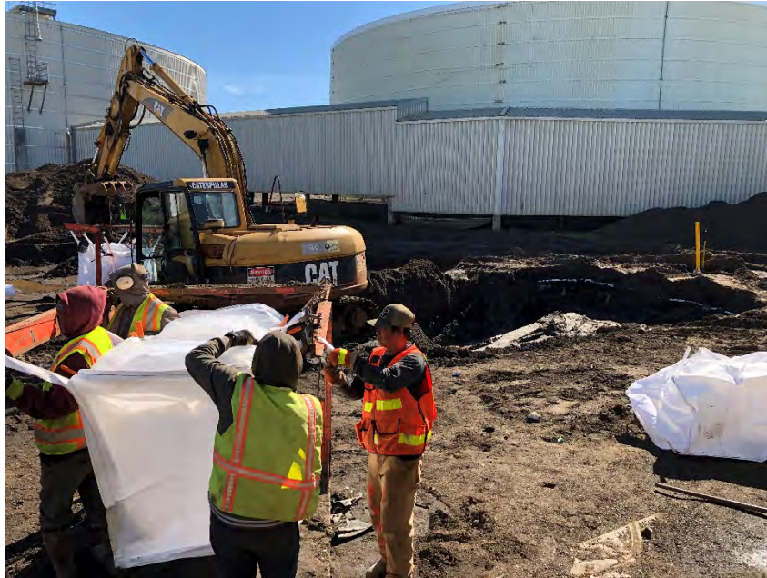
Photograph 1: Containerizing soil excavated from within the hotspot identified on 8/03/21.
