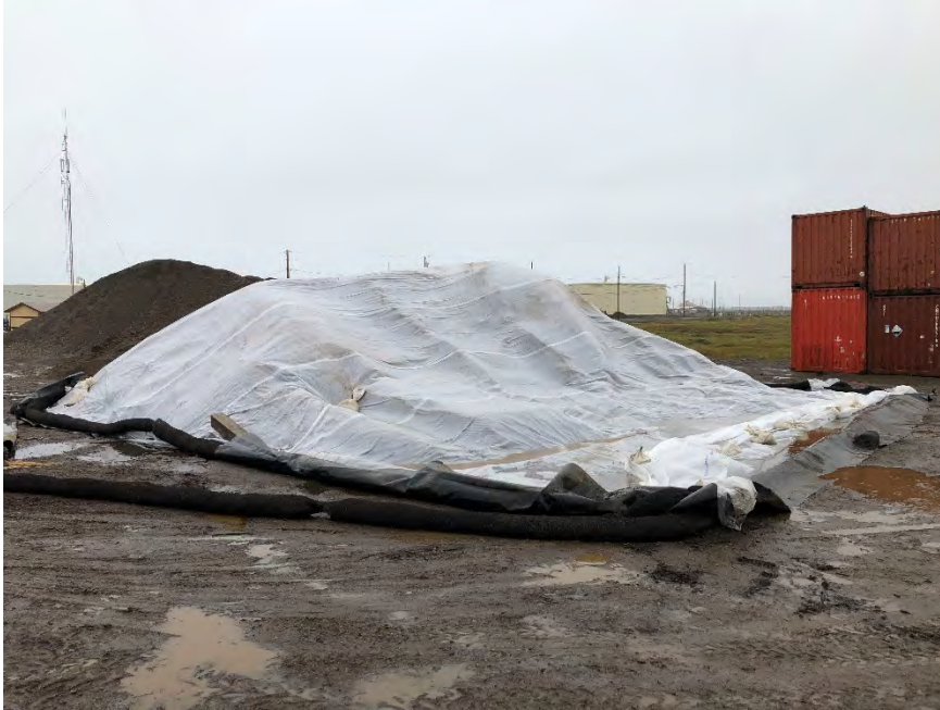
Photograph 2: The potentially clean soil stockpile at the old airport.
