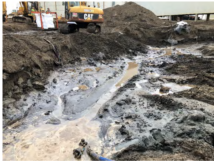
Photograph 3: Pumping the potentially contaminated water into the onsite containment pond.
