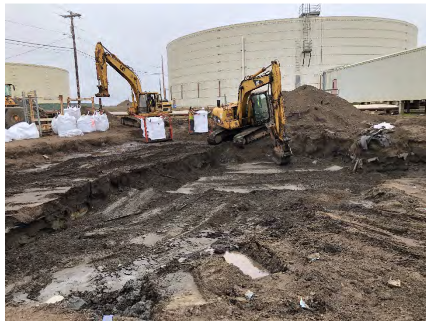
Photograph 4: Excavation and containment of contaminated soil resumed following dewatering.
