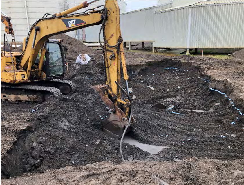
Photograph 1: Excavating and containerizing soil from below 2' bgs exhibiting elevated PID readings.
