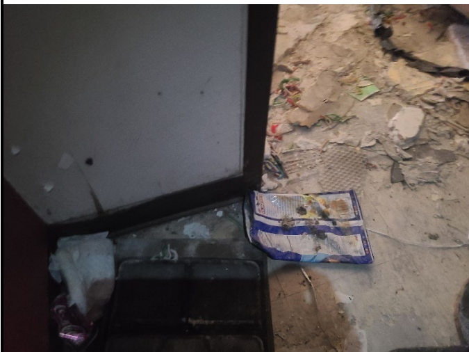
Photo 5. PCBs-containing cove base in Kitchen – Sample PCB09
