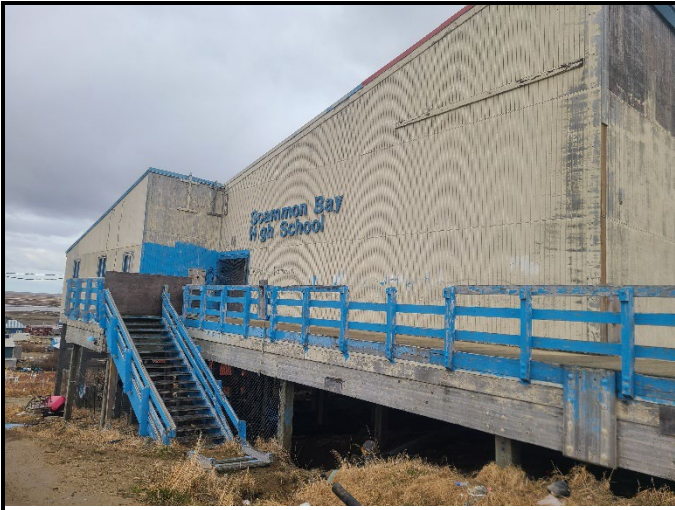
Photo 1. Former Scammon Bay Bureau of Indian Affairs High School; looking north
