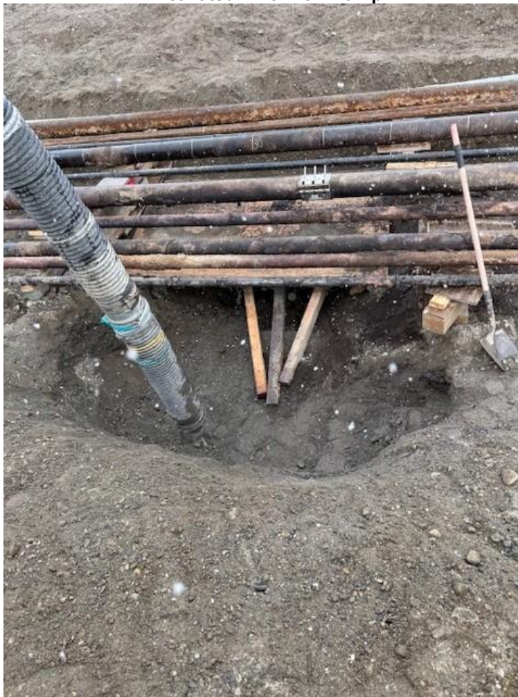
Excavated Line with Clamp
