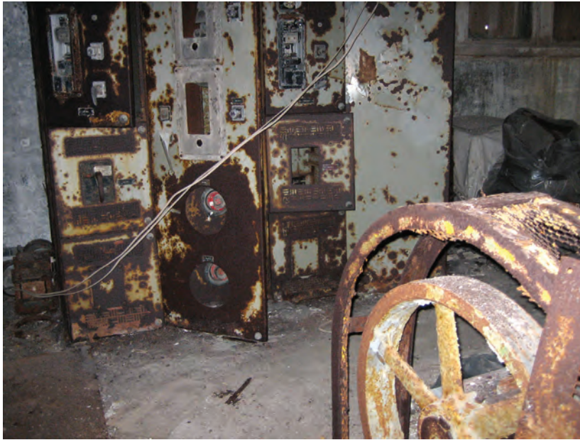
Interior view of the LORAN A Station. D.Rudis, USFWS
