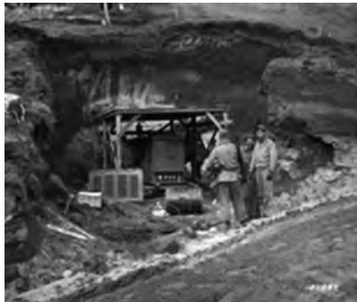
Generator site, Kiska, 1943. U.S. Signal Corps photo
