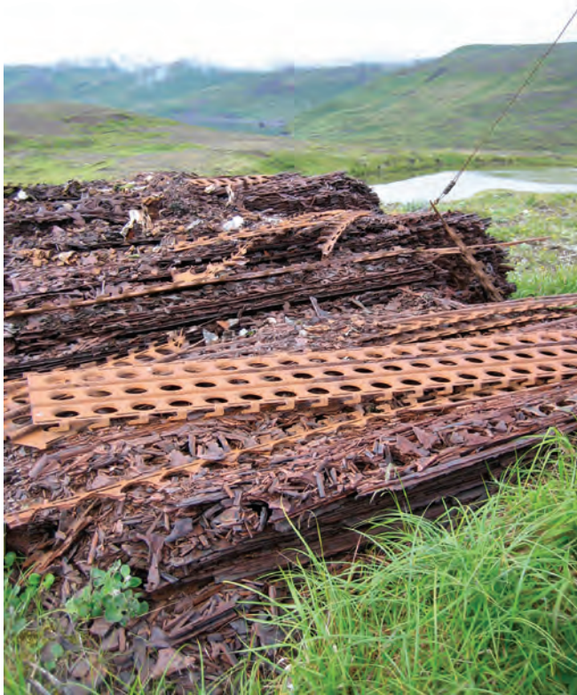
Piles of rusted Marston mat that was used for WWII runway surfacing by U.S. forces are found on Kiska. D. Rudis, USFWS
