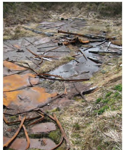
Collapsed tanks at fuel tank farm 2 and residual POL. D. Rudis, USFWS.
