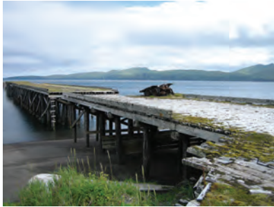
Creosote treated pilings on the Kiska dock. D. Rudis, USFWS
