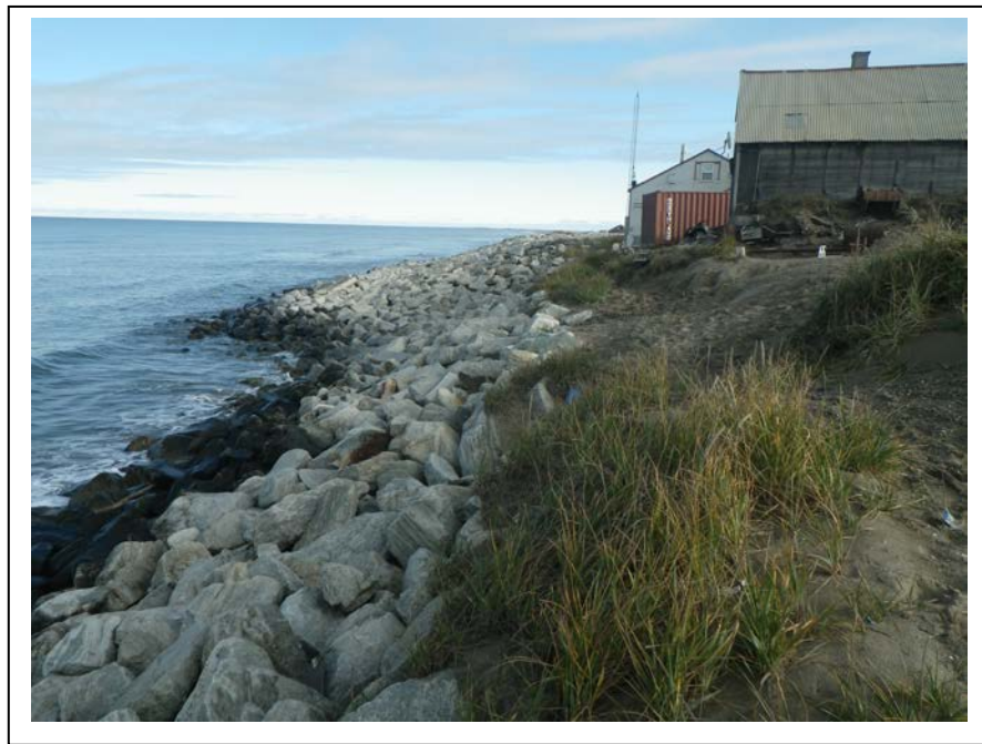
Photo 2: Looking east showing the revetment north of the Warehouse. (September 27, 2018)
