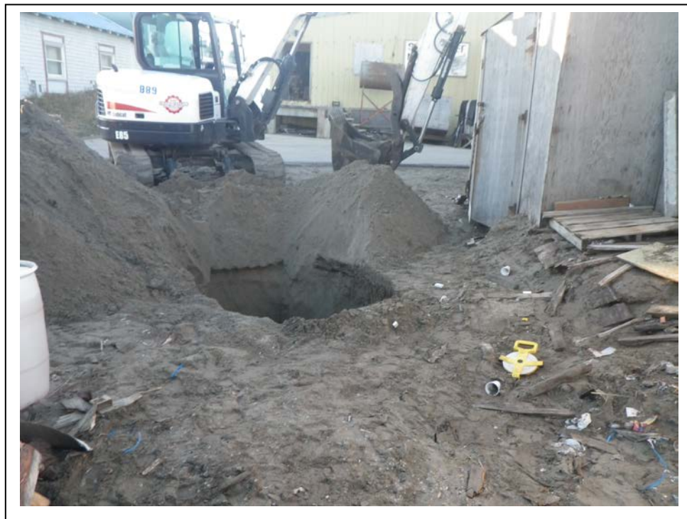
Photo 4: Looking south at Test Pit TP2. (September 26, 2018)
