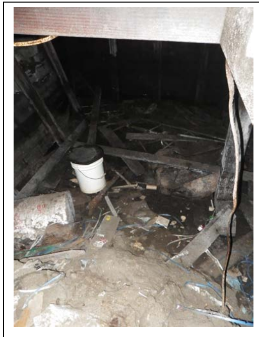
Photo 8: Looking into the cellar beneath the Warehouse. (September 26, 2018)
