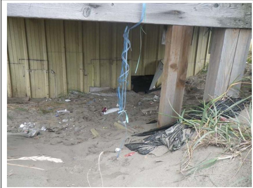
Photo 9: Looking north at the Shishmaref Native Store foundation. (September 26, 2018)
