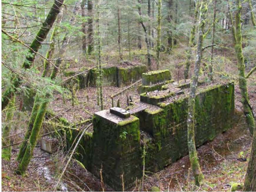
Foundations from Treadwell Hoist, November 2009 Photo Courtesy of Wayne Jensen
