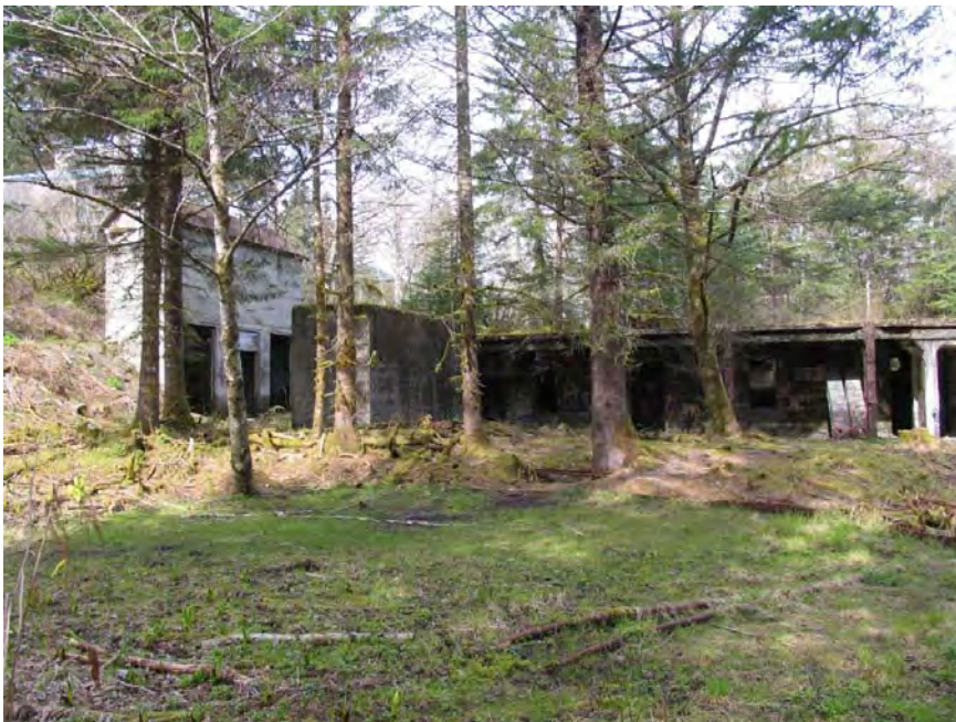
Remains of Central Power Plant, August 2009 Photo courtesy of Wayne Jensen
