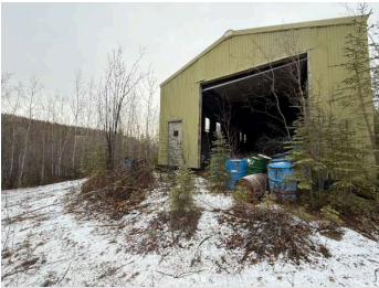
The outside of the warehouse structure. View to the E. (15OCT2025)
