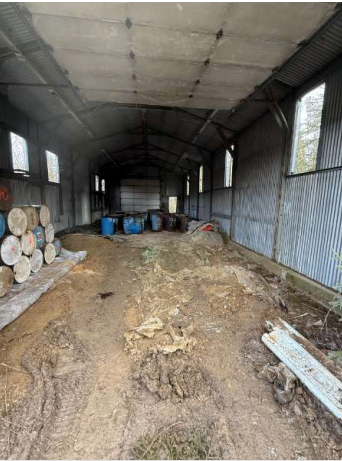
Inside of warehouse at the completion of project. Empties stacked on the left with liquids and solids organized from left to right within the containment area at the back of the warehouse. View looking SE from the open northern door. (17OCT2025)
