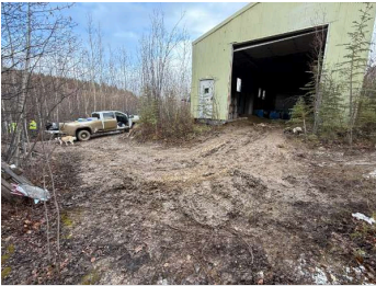
The outside of the warehouse at the completion of project. View looking E. (17OCT2025)
