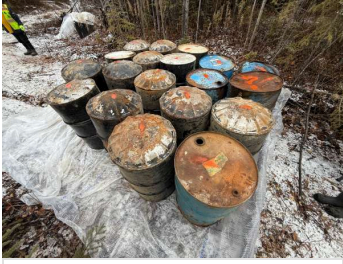
Temporary liner for storage of drums during repositioning. View to the W. (15OCT2025)
