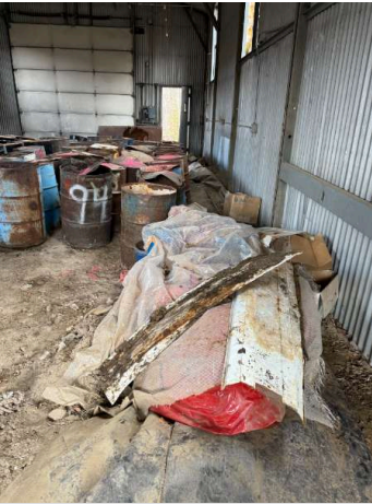
Decaying oily waste bags were consolidated and covered to help preserve brittle plastic bags. View looking S. (17OCT2025)
