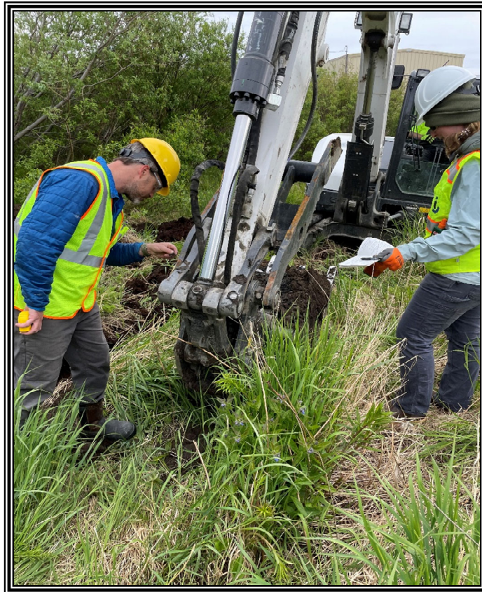
Photograph 1 Logging TP-01. View to the NE. 22JUN23
