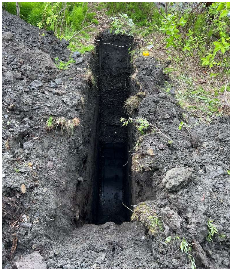
Photo 4. Test pit TP2, which exhibited a petroleum hydrocarbon odor, soil staining, a sheen on perched subsurface water, and free product at the fill-silt interface.
