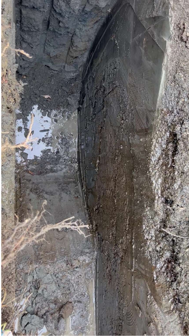
Photo 8. Test pit TP5 with minor accumulation of subsurface water. Petroleum hydrocarbon product is visible along the wall of the test pit at the fill-silt interface. June 23, 2023.
