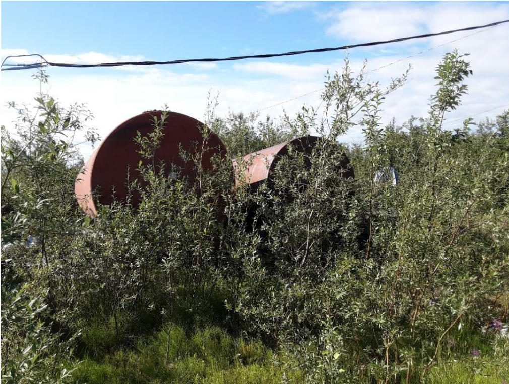
large ASTs, 30-40 ft long, 12-15 ft diam, some rust
