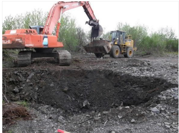
Photo 4: Initial Site excavation in 2012
