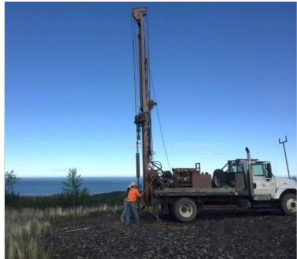
Photo 5: Drilling monitoring wells at the Site
