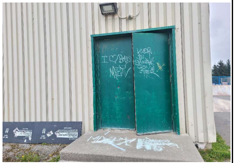
Photo 14. LBP Reading #640; Building 1 S.W. Entrance.
