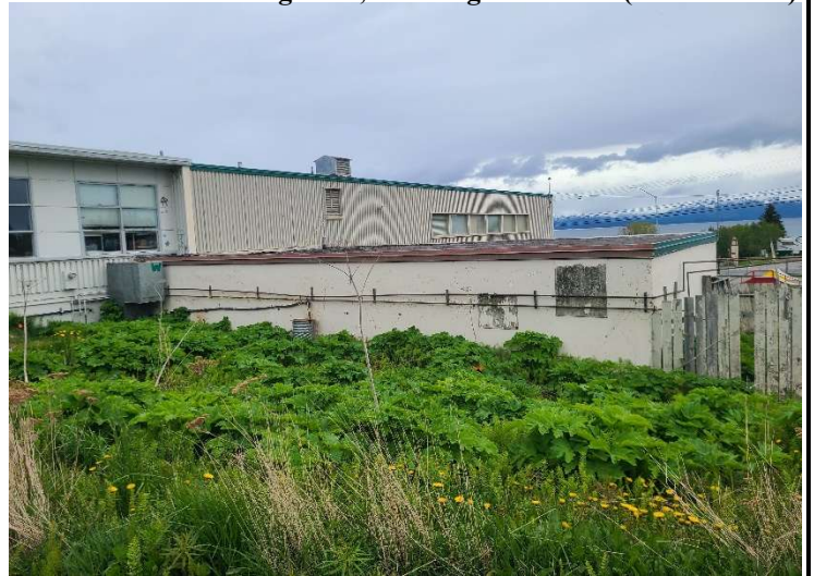
Photo 10. Building 1 Western Extension (Looking South).
