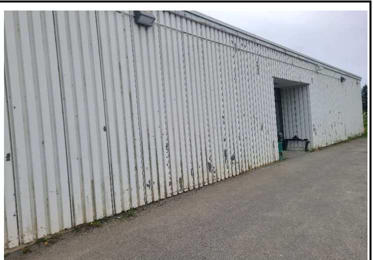
Photo 8. LBP Reading #620; Building 1 Exterior (Lookin S.W.).
