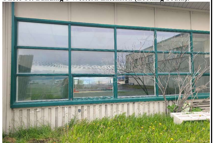
Photo 12. LBP Reading #633; Western Extension Window.
