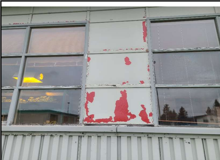
Photo 7. LBP Reading #617; Building 1 Exterior.
