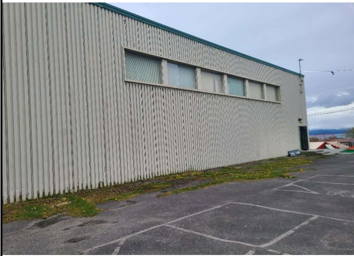
Photo 13. LBP Reading 638; W. Exterior Bldg. 1 (Looking S.).
