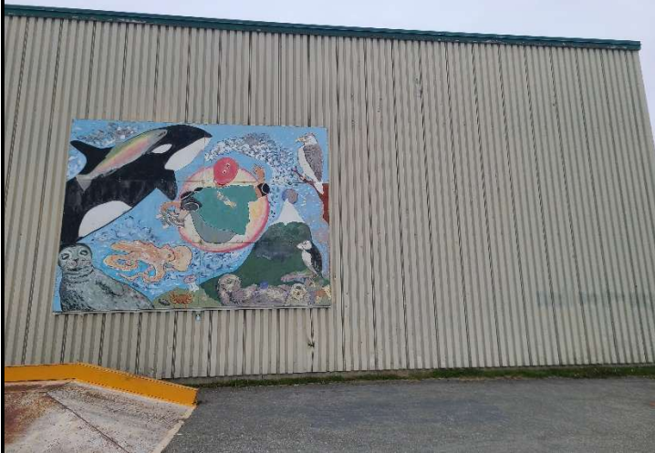
Photo 15. LBP Reading #642; Bldg. 1 South Exterior Wall.
