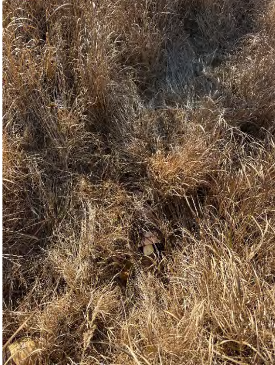
Photograph 45: OT001, subarea PT1, destroyed monitoring well along trail through PT1, view down. 9/24/2025
