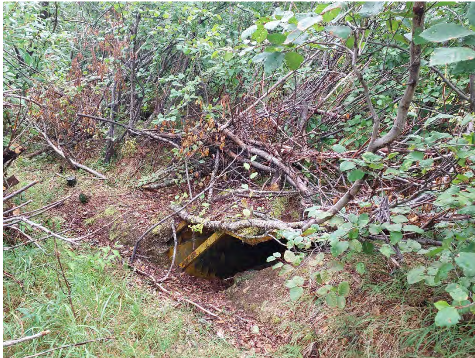
Photograph 16: LF002, subarea LF1, buried heavy equipment, view southwest. 8/22/2025
