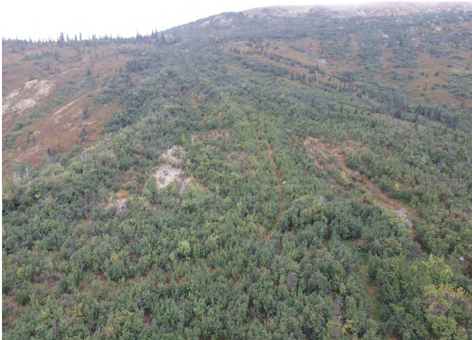
Photograph 20: Aerial overview of LF002, subarea LF2, view south. 8/22/2025
