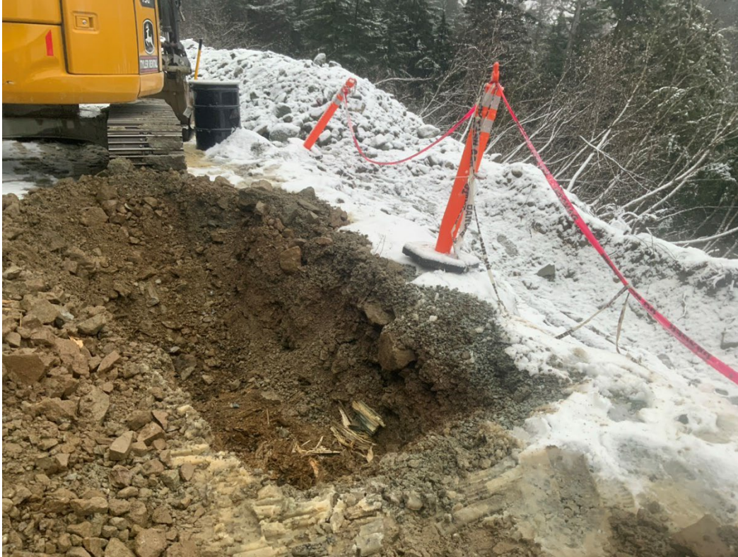
7. Looking Northeast, showing the eastern sidewall of pothole SB02.
