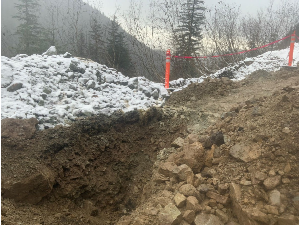
15. Looking Southeast, showing the eastern sidewall of pothole SB09.
