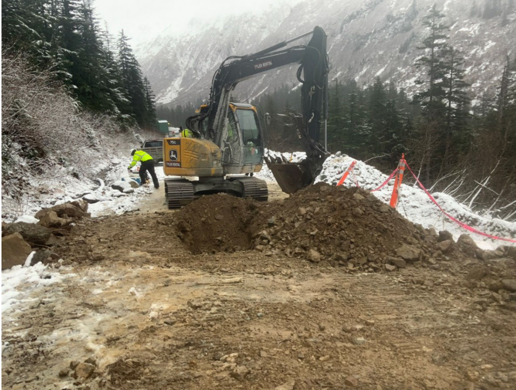
13. Looking North, showing the excavation location of pothole SB08.
