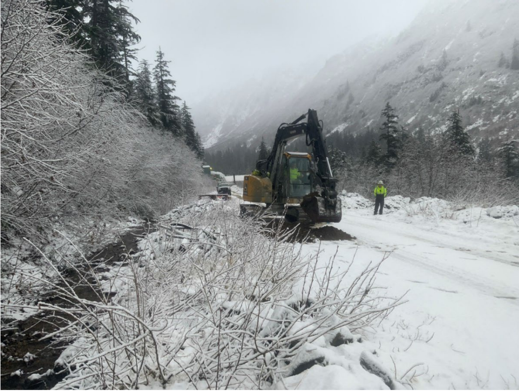
1. Looking North, along Pipeline Road showing excavation location of BG01.
