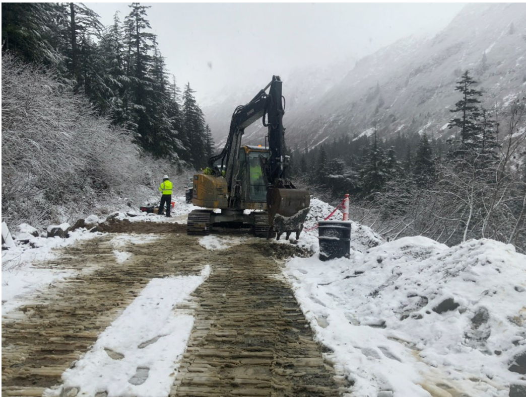
4. Looking North, along Piepline Road showing excavation location of pothole BG01.
