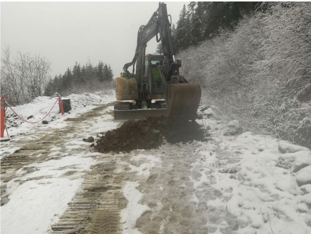
2. Looking South, along Pipeline Road showing excavation location of BG02.
