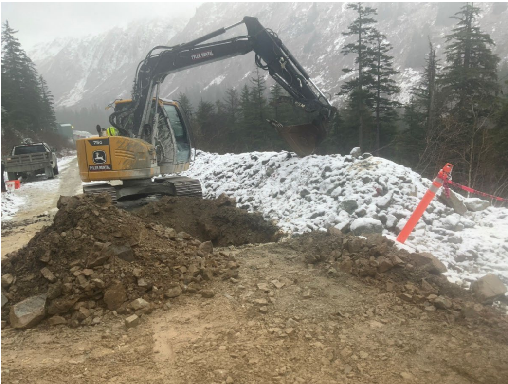
14. Looking Northeast, showing the excavation location of pothole SB09.
