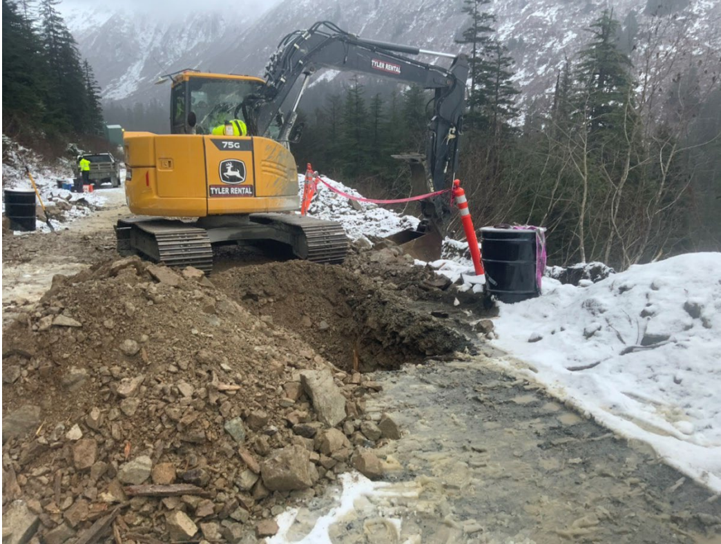
11. Looking Northeast, showing the excavation location of pothole SB07.
