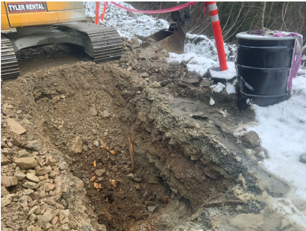
12. Looking Northeast, showing the eastern sidewall of the pothole SB07.
