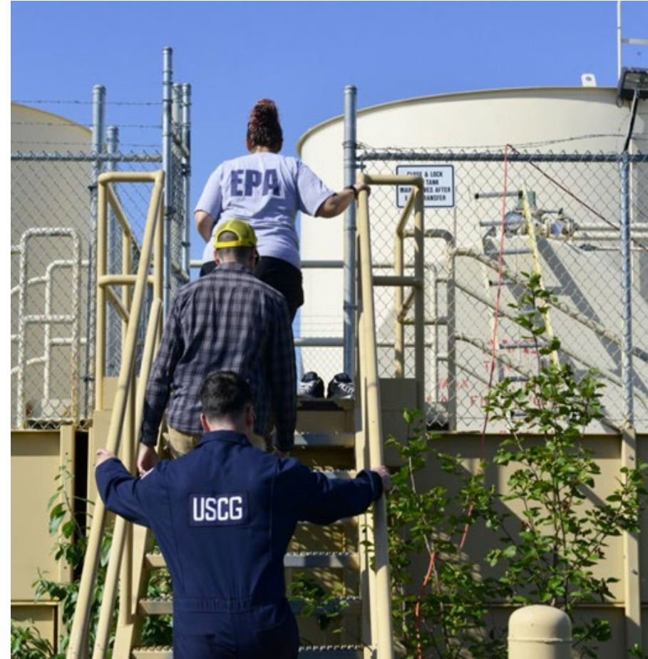
2022 USCG & EPA conduct joint inspections in Selawik
