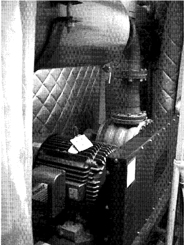
The new 40-horsepower Roots® rotary-lobe air blower at the University of Alaska Fairbanks that powers the 49-diffuser aerator array.
