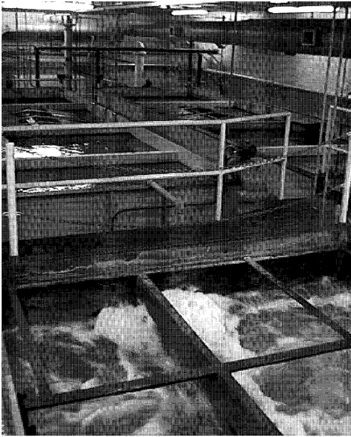
The UAF water treatment plant. In the foreground, froth forms on the water being agitated in the aerator. Behind the aerator are the two sets of two flocculation tanks, the sedimentation tanks with their submerged tube settlers, and the filter tanks at the end of the treatment line.
