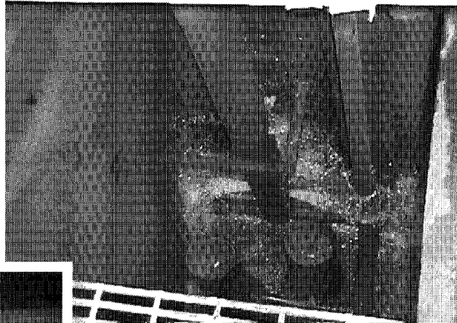
Aerator basin at UAF, beginning to refill with water after cleaning the basin and diffusers.
