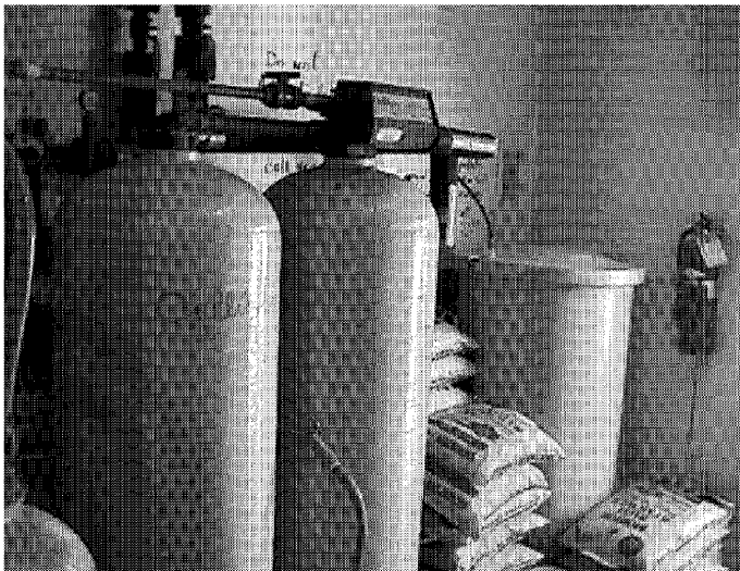
Water softeners and bags of rock salt for resin regeneration at a Fairbanks business establishment.
