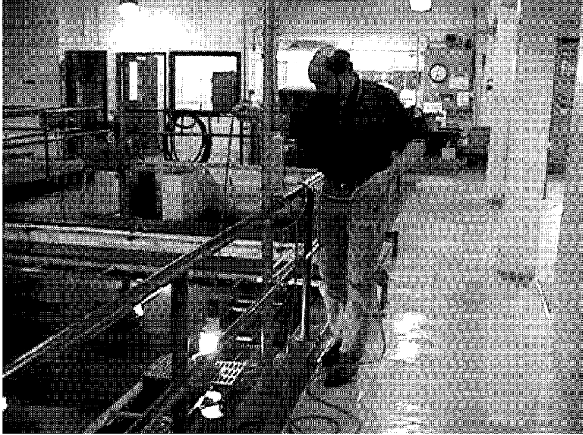
Measuring the depth of the floc blanket at the Golden Heart Utilities water treatment plant in Fairbanks, Alaska. The operator lowers a lamp into the clarifier until the light is obscured by the layer of floc.
