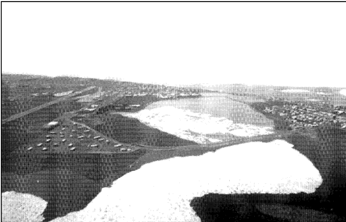
Barrow, Alaska, showing the Isatkoak Reservoir (water body in the foreground), separated by the Isatkoak Lagoon by the Isatkoak Dam (running horizontally through the center of the photograph). The Arctic Ocean is on the horizon, and the small Tasigarook Lagoon lies between the ocean and Isatkoak Lagoon. The Barrow Utilities and Electric Cooperative, Inc., water treatment plant lies on the upper, left-hand shore of Isatkoak Lagoon.
