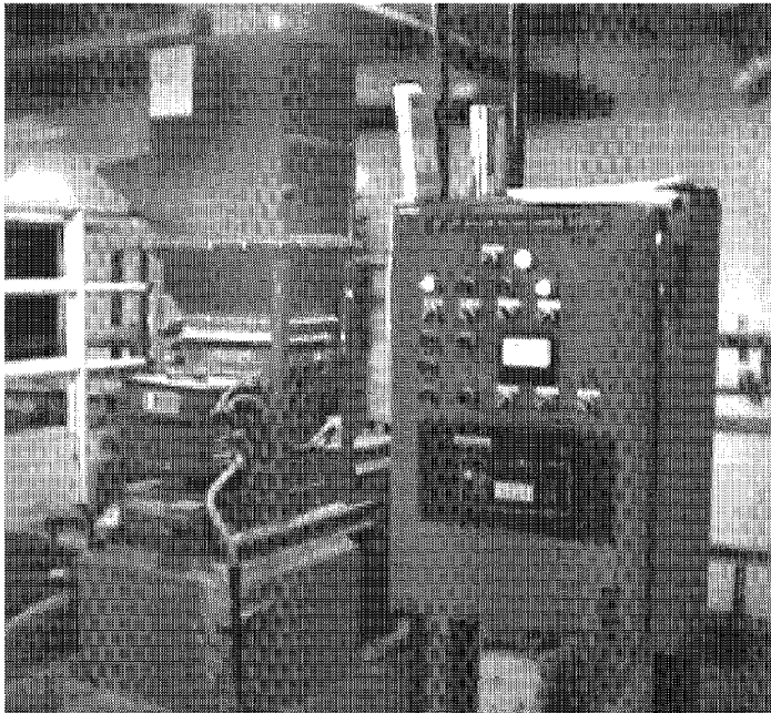
Dry chemical volumetric feeder and controls for feeding sodium fluorosilicate at the Golden Heart Utilities Water Treatment Plant in Fairbanks, Alaska.
