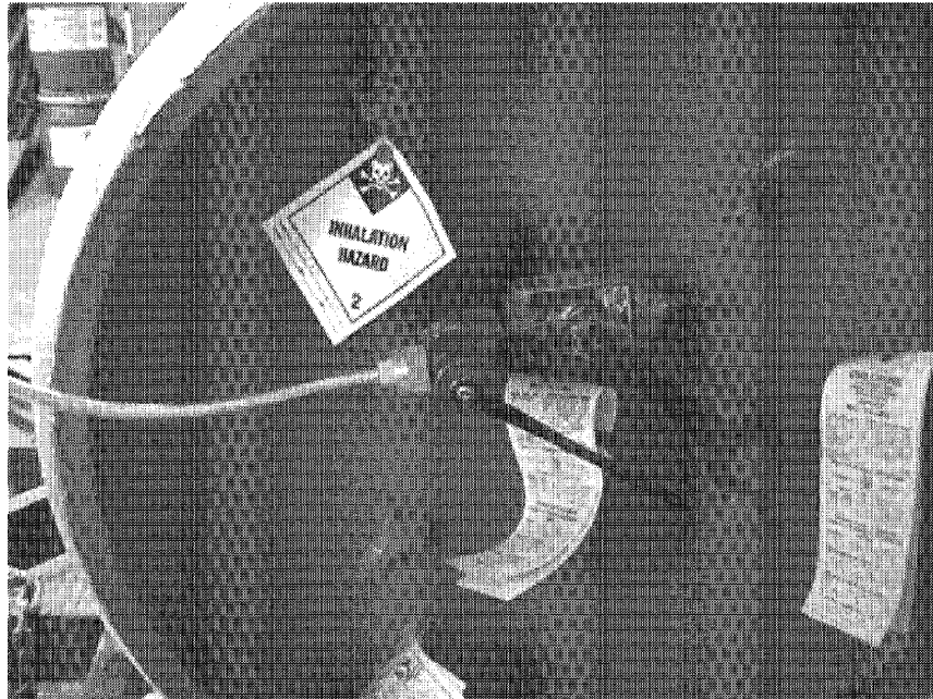
Close-up of top of ton chlorine gas container, showing wrench on control valve.
