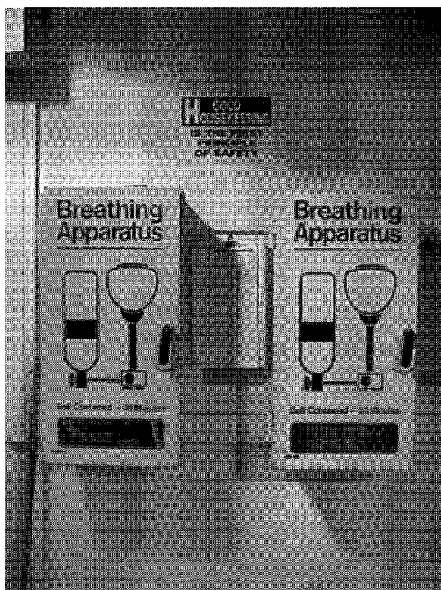
Self-contained breathing apparatus boxes just outside the gas chlorine room at the Golden Heart Utilities water treatment plant, Fairbanks, Alaska.
