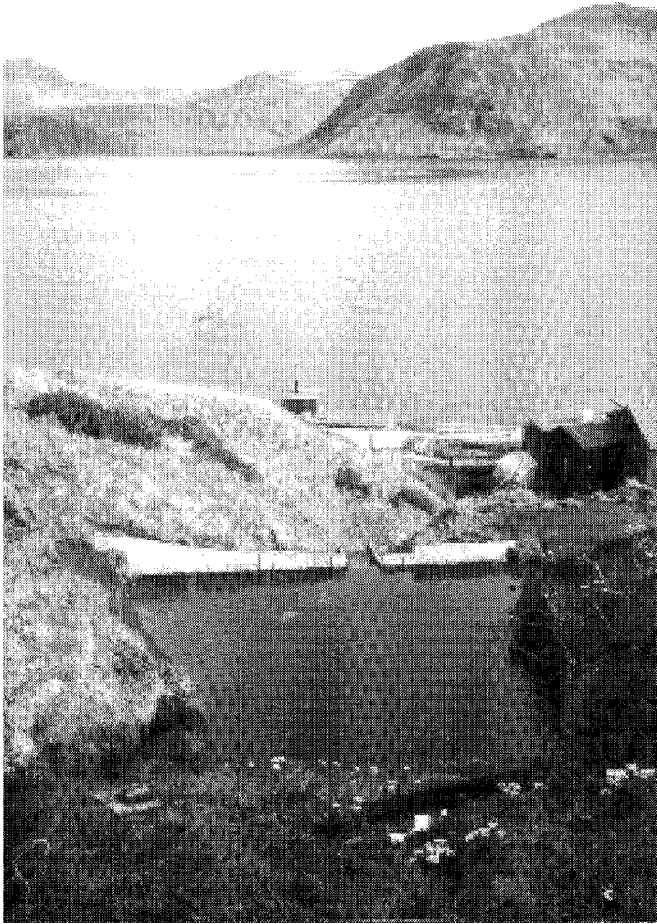
Surface water catchment for the Village of Akutan in the Aleutian Islands. The catchment's wooden dam is equipped with a high water overflow (center).
