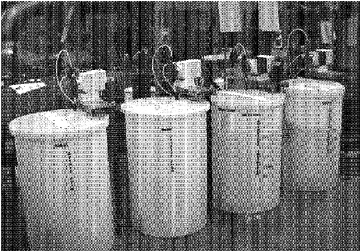
Chemical feed stations at the Barrow Utilities and Electric Cooperative, Inc., water treatment plant.
