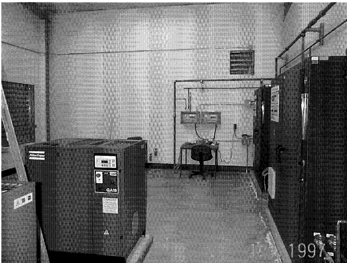
The ozone generators and associated air compressors at the City of Wrangell Water Treatment Plant. Photo courtesy of the City of Wrangell Water Treatment Plant and Greg Scheff and Associates.
