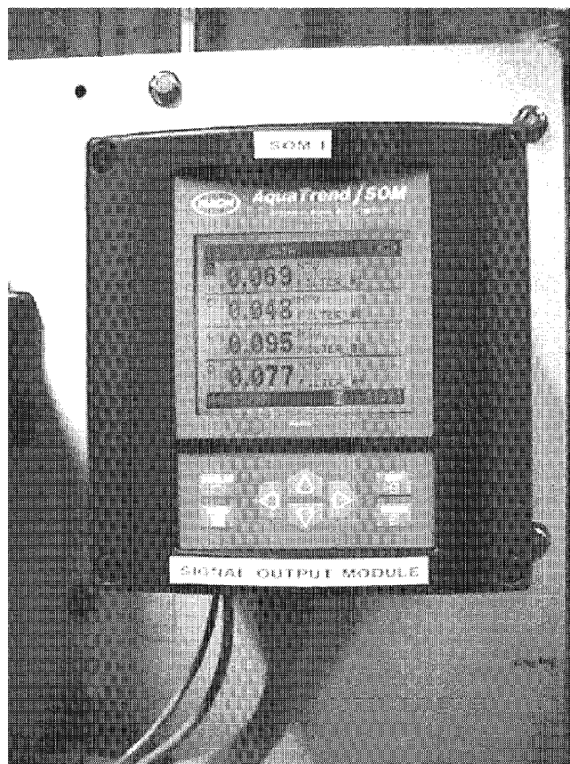
Hach Aquatrend® Interface datalogger, Ship Creek Water Treatment Facility, Anchorage, Alaska. This instrument records data from the on-line turbidimeters and particle counters that monitor the four filters at the treatment plant.
