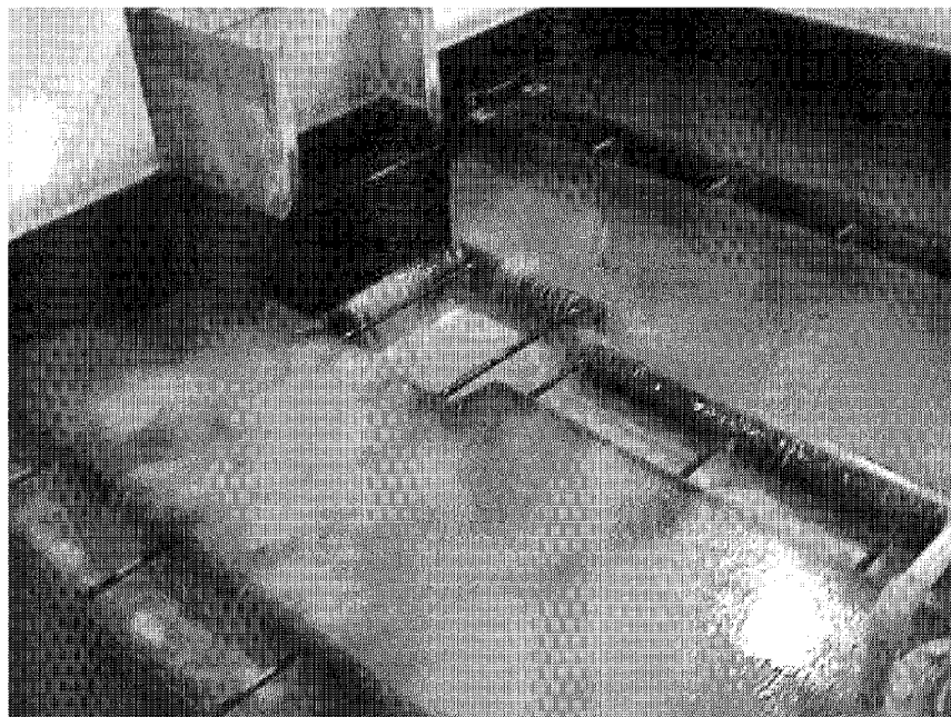
Continuation of backwashing sequence at Golden Heart Utilities. Top: water continuing to rise up through the filter. Bottom: backwash water overflowing into the wash-water troughs.
