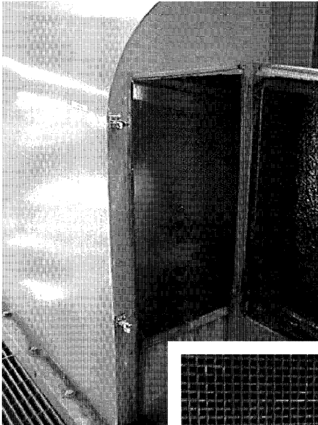
Traveling screen at the Ship Creek Water Treatment Facility in Anchorage, Alaska. Counter-clockwise from top: Wire-mesh screen housing; looking inside the housing; close-up of wire mesh.
