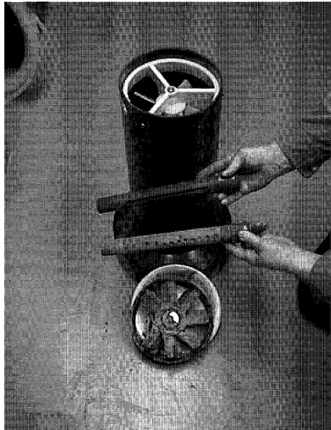
New Ramco® air diffuser and used diffuser encrusted with iron precipitates. The new slitted blow-tube replaces encrusted tube with holes drilled in it.
