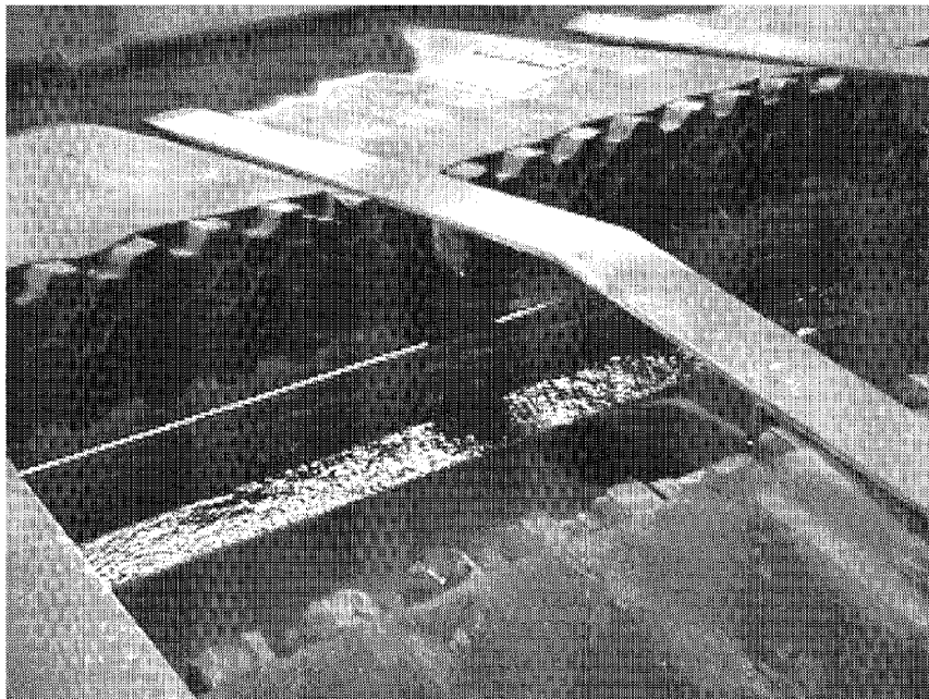
Above: The sedimentation basin at the University of Alaska Fairbanks. Tube settlers are submerged in the basin at a 15° angle. Below: Detail of the hexagonal tube settlers in their honeycomb arrangement inside the sedimentation basin.
