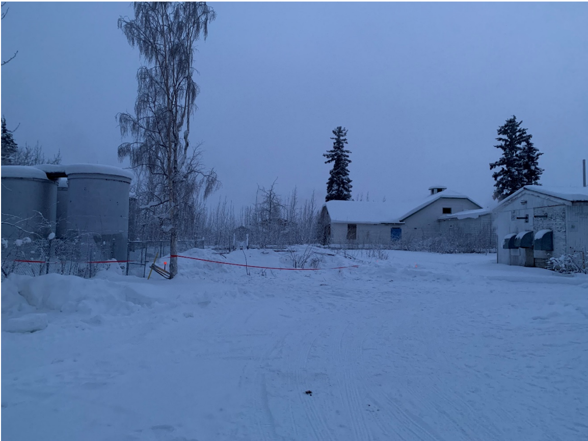
Spill area looking south, with school tank farm on the left and generator shack on the right. Affected line visible on top of snow pile.
