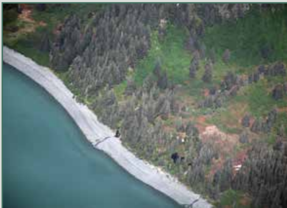
PR01 & DAM-U02 viewed from the southwest.
