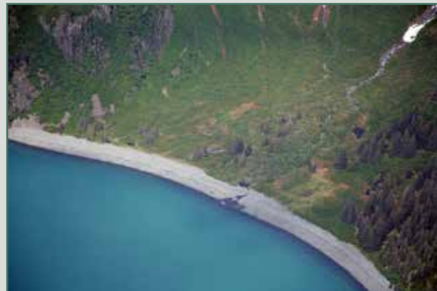
DAM-U02b viewed from the southwest.
