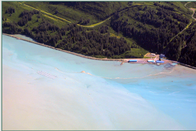
PWS NE13-02 Solomon Gulch Hatchery looking southeast.
