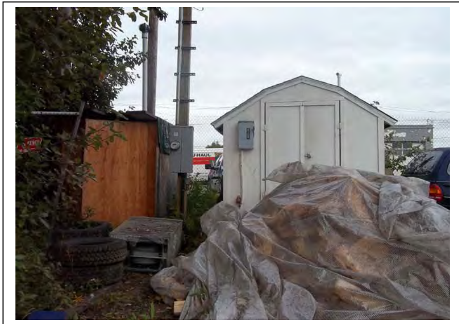
Photo 28: Two outbuildings are located north of the 3609 Spenard Road structure; looking west. (August 17, 2012)
