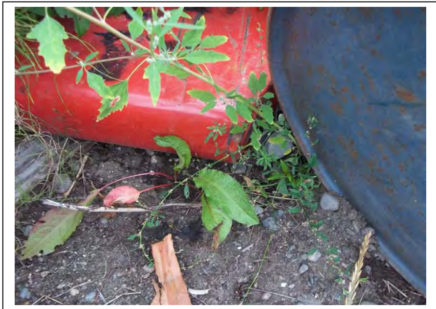
Photo 18: Surface staining was observed near the overturned drums and fuel container. (August 17, 2012)
