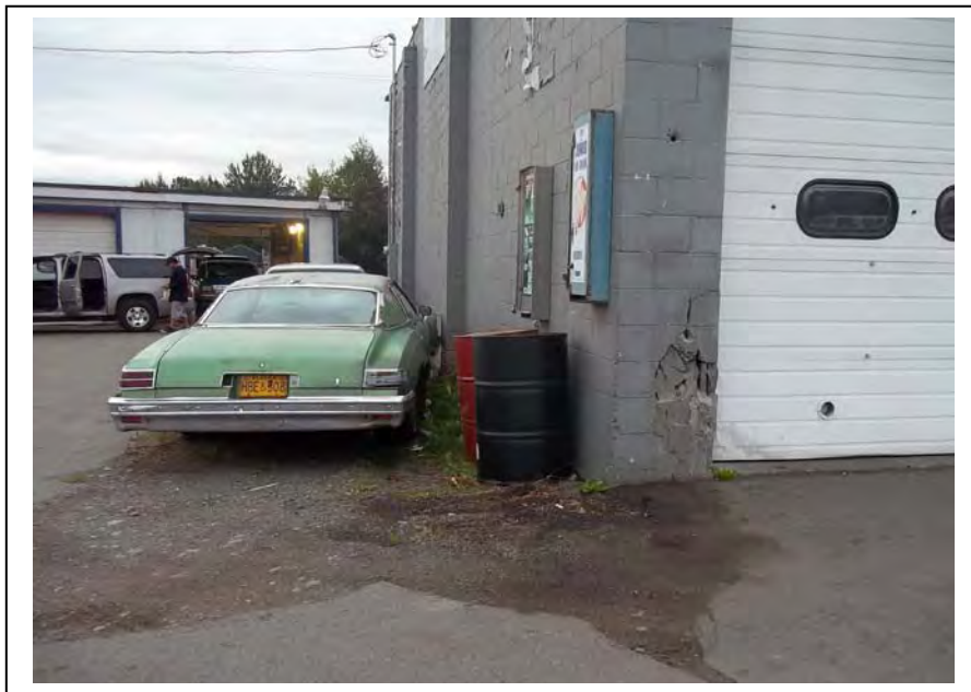
Photo 12: Two empty 55-gallon drums were observed near the northeast corner of the Alpina Auto Repair structure; looking east. (August 17, 2012)
