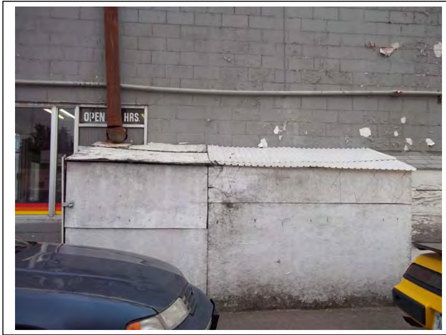
Photo 13: A storage shed is located adjacent to the south wall of the Alpina Auto Repair structure; looking north. (August 17, 2012)
