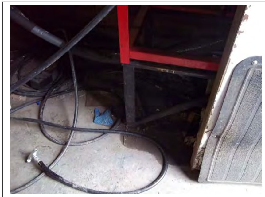
Photo 10: Surface stains were observed in the eastern storage room of the car wash structure. (August 17, 2012)
