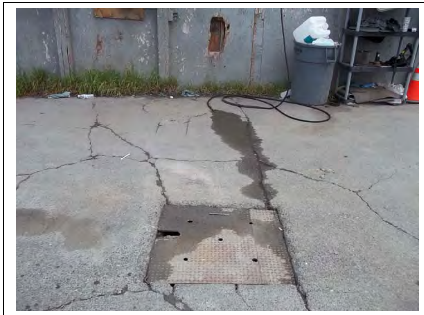
Photo 8: Exterior drain and possible sand trap or oil/water separator; looking north. (August 17, 2012)
