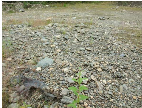
Photo 12: Looking southeast, liner was observed along the edge of the gravel fill material. (Waypoint 82, 8/15/2012)
