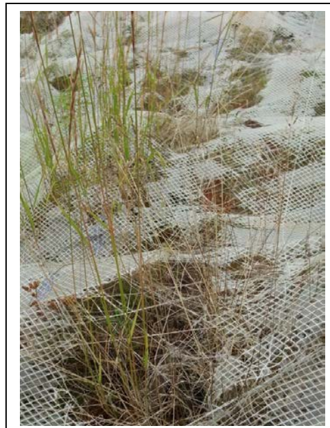
Photo 2: The top cover of the stockpile appeared weathered and was deteriorating. (Waypoint 59, 8/15/2012)
