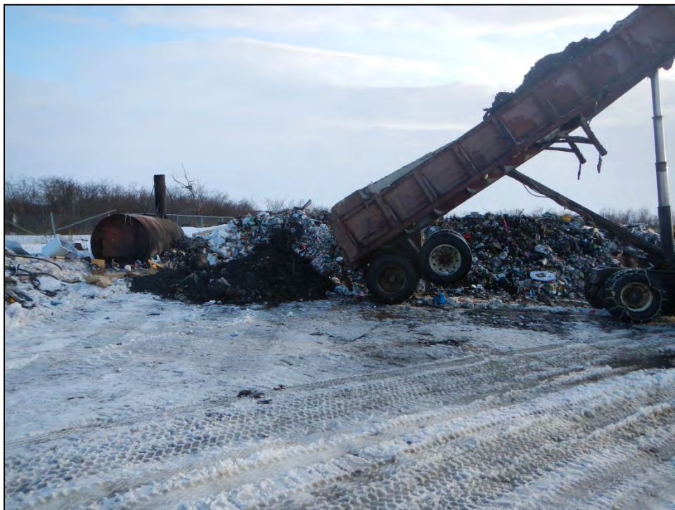
PHOTOGRAPH 6: DUMPING DEBRIS/SOIL AT KWETHLUK DUMP (LOOKING SOUTH).
