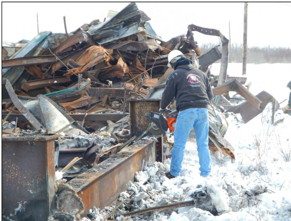
PHOTOGRAPH 4: CUTTING BEAMS AWAY FROM STEEL PILES (LOOKING SOUTH).
