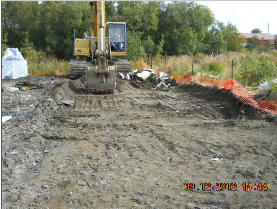
PHOTOGRAPH 15: SEPTEMBER 2012 EXCAVATION AROUND LOCATIONS A5, B5, AND C5 (LOOKING EAST).
