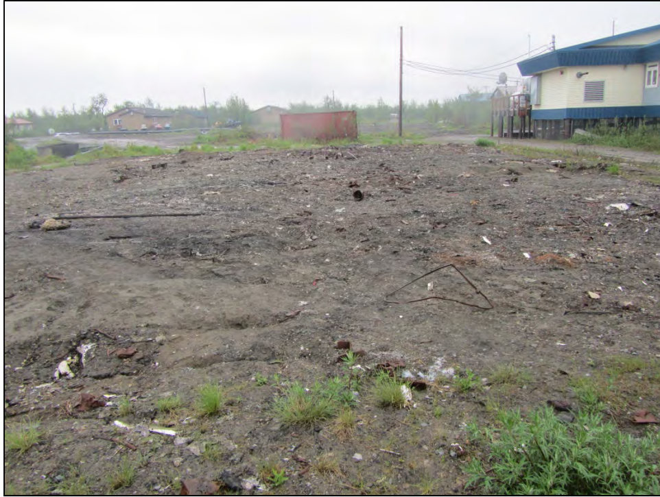
PHOTOGRAPH 7: BUILDING FOOTPRINT AFTER SPRING FLOODING AND BEFORE DEBRIS CLEANUP (LOOKING SOUTH).
