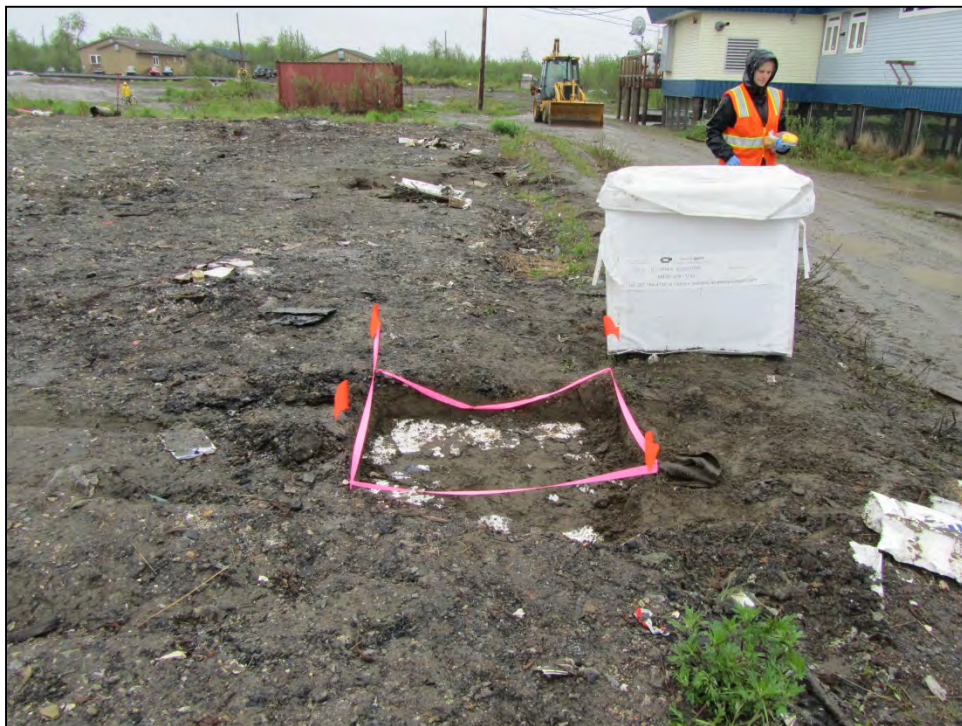
PHOTOGRAPH 12: EXCAVATION AREA 2 WITH BULK SACK - JUNE 2012 (LOOKING SOUTH).
