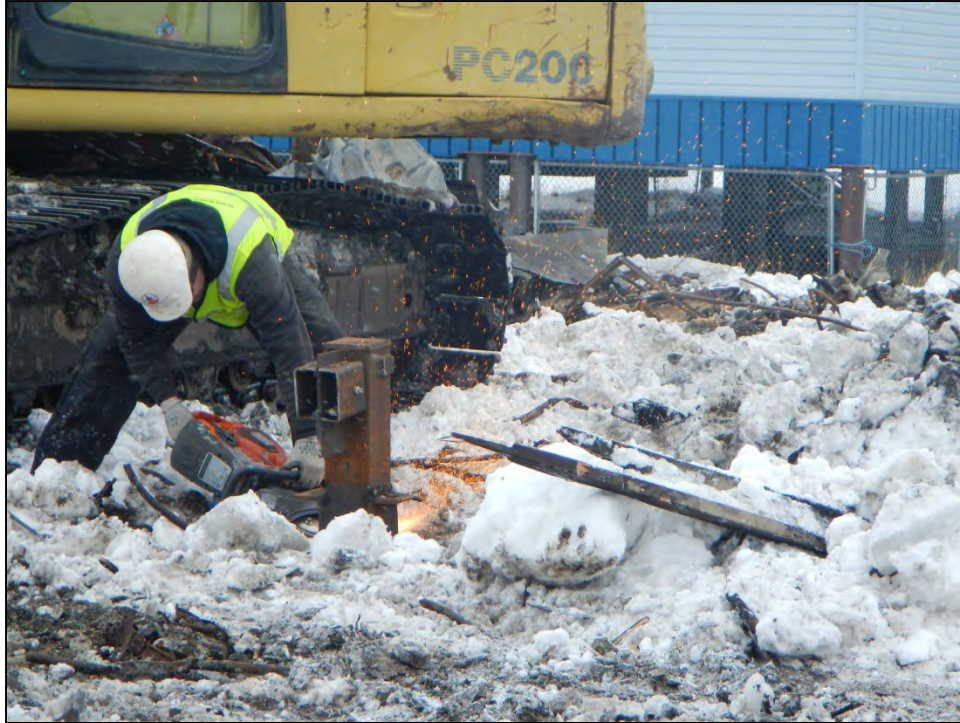
PHOTOGRAPH 5: CUTTING VERTICAL PILES BELOW GRADE (LOOKING WEST)
