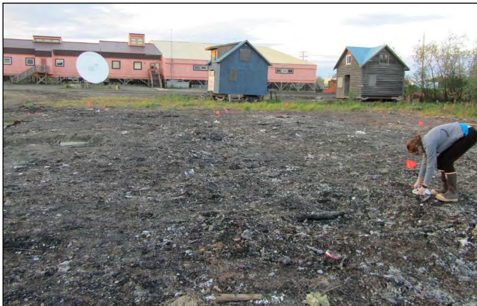
PHOTOGRAPH 8: BUILDING FOOTPRINT AFTER METAL CLEANUP (LOOKING NORTH).
