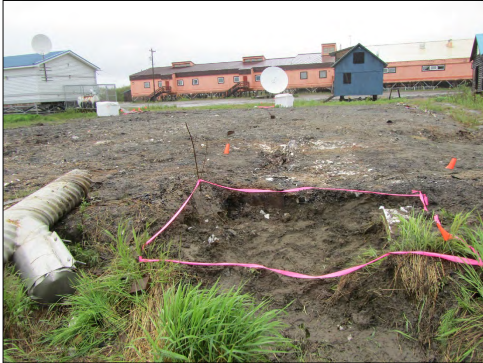
PHOTOGRAPH 11: EXCAVATION AREA 1 - JUNE 2012 (LOOKING NORTH)
