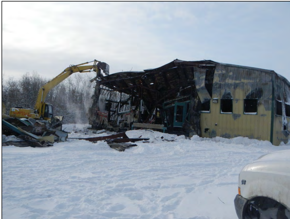
PHOTOGRAPH 1: DISMANTLING THE FRAME AND STRUCTURE OF THE JGCC BUILDING (LOOKING SOUTH).
