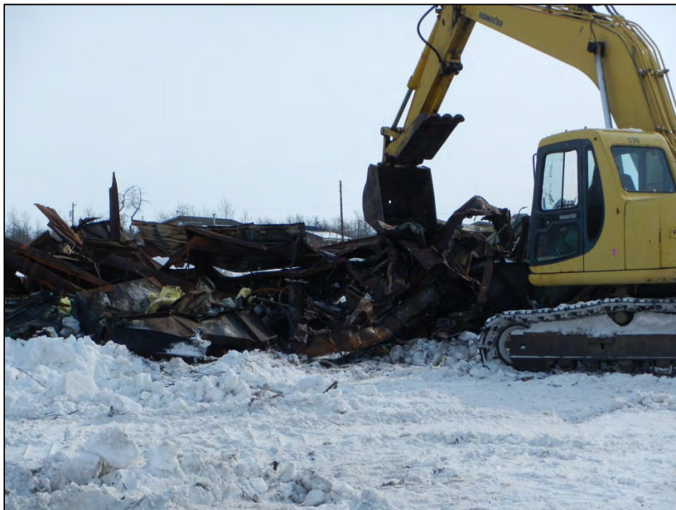
PHOTOGRAPH 2: STAGING AND CRUSHING METAL DEBRIS FOR TRANSPORT TO BETHEL LANDFILL (LOOKING SOUTHEAST).
