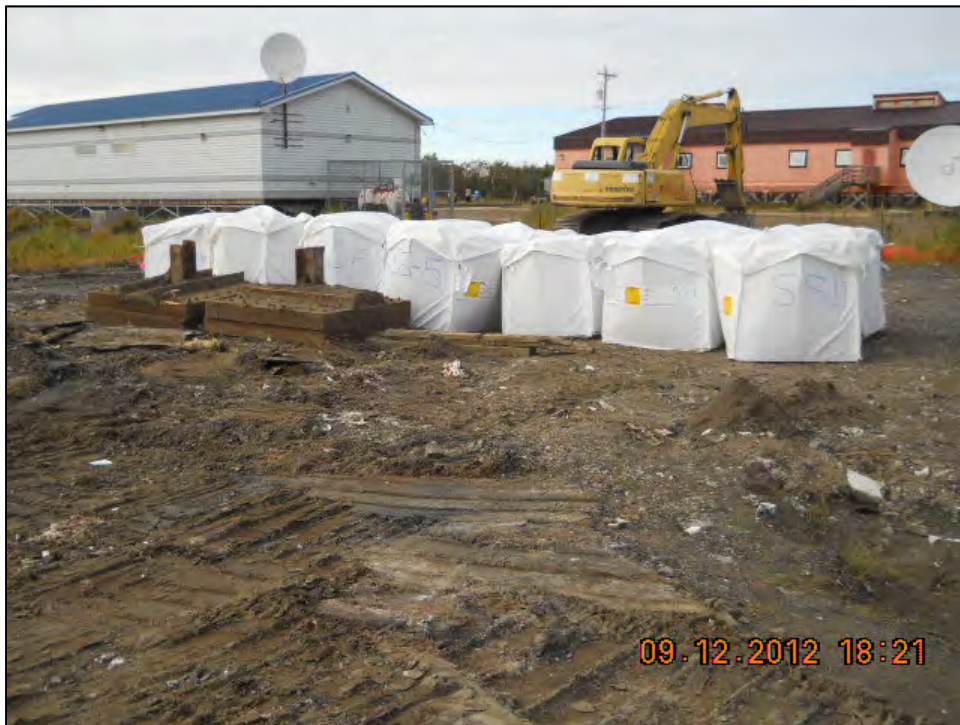
PHOTOGRAPH 16: STAGING LOCATION FOR BULK SACKS AND PILING PENDING ANALYTICAL RESULTS (LOOKING SOUTHWEST).
