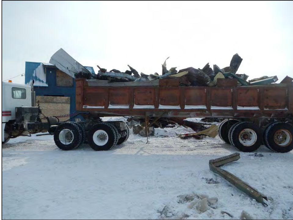
PHOTOGRAPH 3: DUMP TRUCK LOADED AND READY TO HAUL ACROSS ICE ROAD TO BETHEL LANDFILL (LOOKING EAST)
