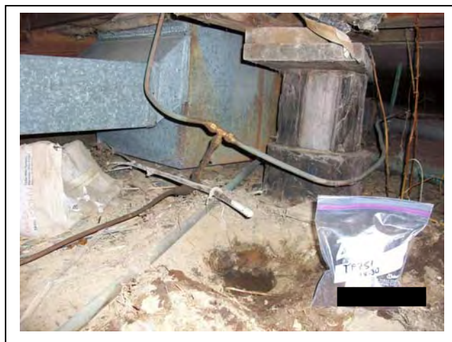
Photo 9: Galvanized duct work for forced-air furnace, copper fuel lines, wood support blocks, and Test Pit TP7 location beneath building, looking southeast 10/25/2010.
