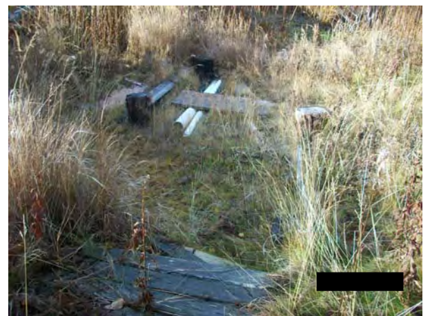
Photo 4: Depression, stressed vegetation, and creosote-treated timber supports thought to be the location of a former electric generator, looking north-northwest 10/25/2010.
