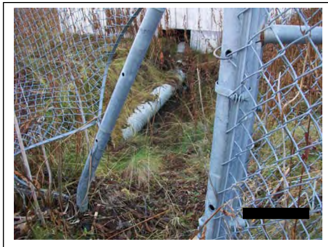
Photo 7: Damaged chain-link fence and exposed, broken sewer line at south end of Old School, looking northwest 10/25/2010.
