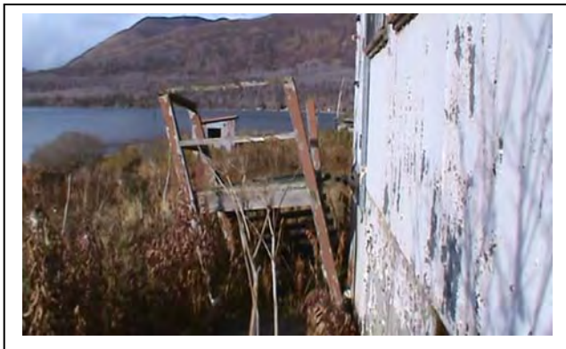
Photo 6: Collapsing stairs at northern Old School entrance, flaking paint, and cement board skirting, looking north-northwest 10/25/2010.
