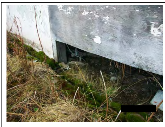
Photo 8: Plywood replacement for cement board skirting at northeast corner of Old School, plastic and galvanized water piping visible under building, looking south 10/25/2010.
