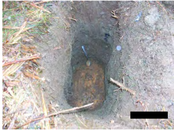
Top of steel underground storage tank located south-southwest of the Old School building, with table spoon for scale, looking south on 10/26/2010.
