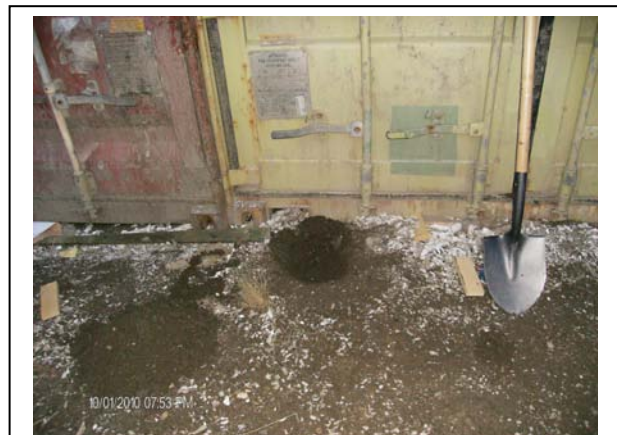
Photograph 5.2-3: Looking north at broken fluorescent bulbs and the Sample BLS2 location at the base of shipping containers on the Barge Landing storage pad. (10/1/2010)
