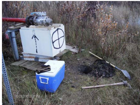
Photograph 5.2-6: Looking northwest toward the marine header, drip tub, and Sample BLS1 location. (10/1/2010)
