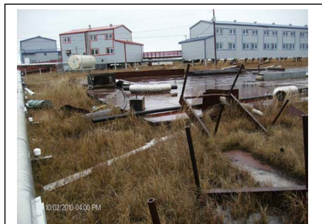
Photograph 7.2-4: Looking south-southwest across the Storage Pad, with piping, construction debris, a drum, and scrap visible. (10/2/2010)
