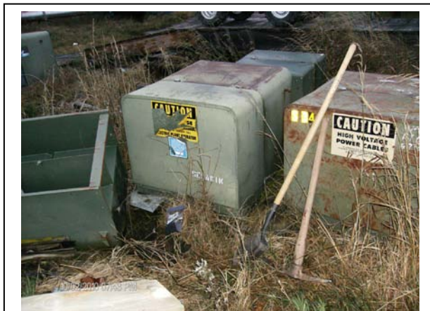
Photograph 6.2-5: Electrical boxes near the southeast corner of the Former AVEC Facility, and the Sample AVS8 location next to the upturned box, looking west-southwest. (10/2/10)
