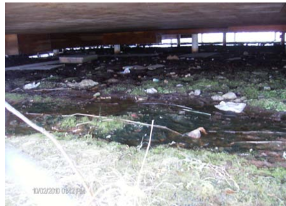
Photograph 7.2-2: Looking northwest beneath the Davis-Ramoth School. Ice and water is visible on the ground surface, which appears to be wet peat with residual tundra vegetation. (10/2/2010)
