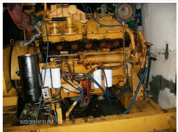
Photograph 6.2-3: One of two diesel engines for electrical generation in the Butler building at the Former AVEC Facility, looking south. (10/2/2010)
