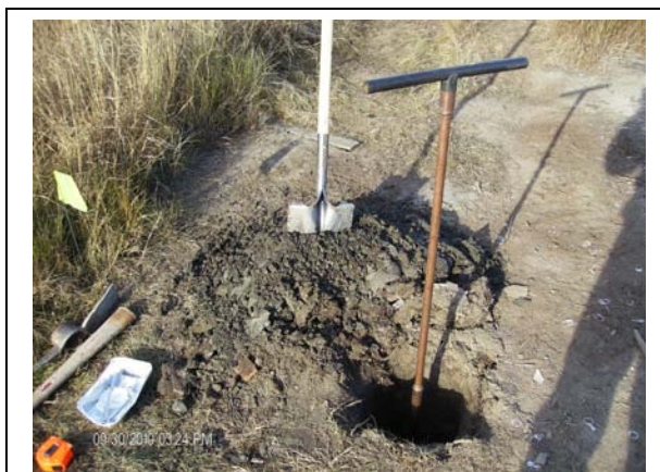
Photograph 4.2-4: Looking down at Test Pit I1 advanced by hand using a shovel and hand auger at the IRA Fuel Project Former Tank Farm. Stained soil associated with the former dispenser shed visible to left. (9/30/2010)
