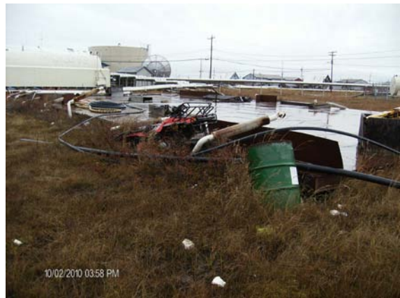
Photograph 7.2-5: Looking southeast at the steel Storage Pad with cooling risers, drum and 4-wheeler in foreground and a fuel tank and water tank in background. (10/2/2010)
