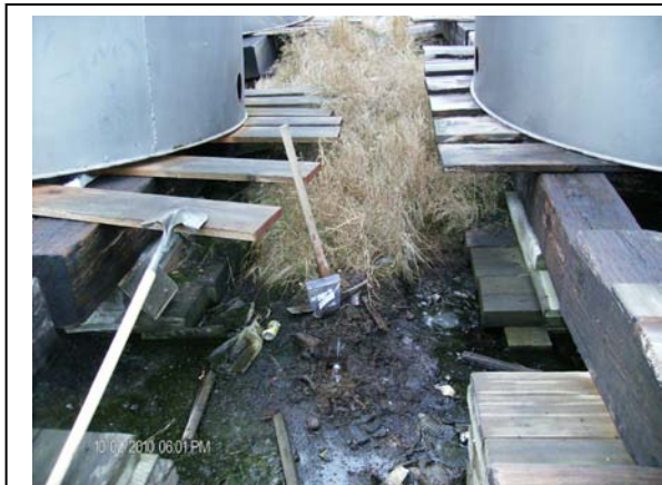
Photograph 6.2-2: Decommissioned ASTs remaining at the Former AVEC Facility, and stained soil at the Sample AVS4 location, looking north. (10/2/2010)
