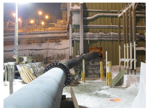
The 24-inch bypass line, under construction, enters the metering building at PS 1. (Photo courtesy of ADEC)
