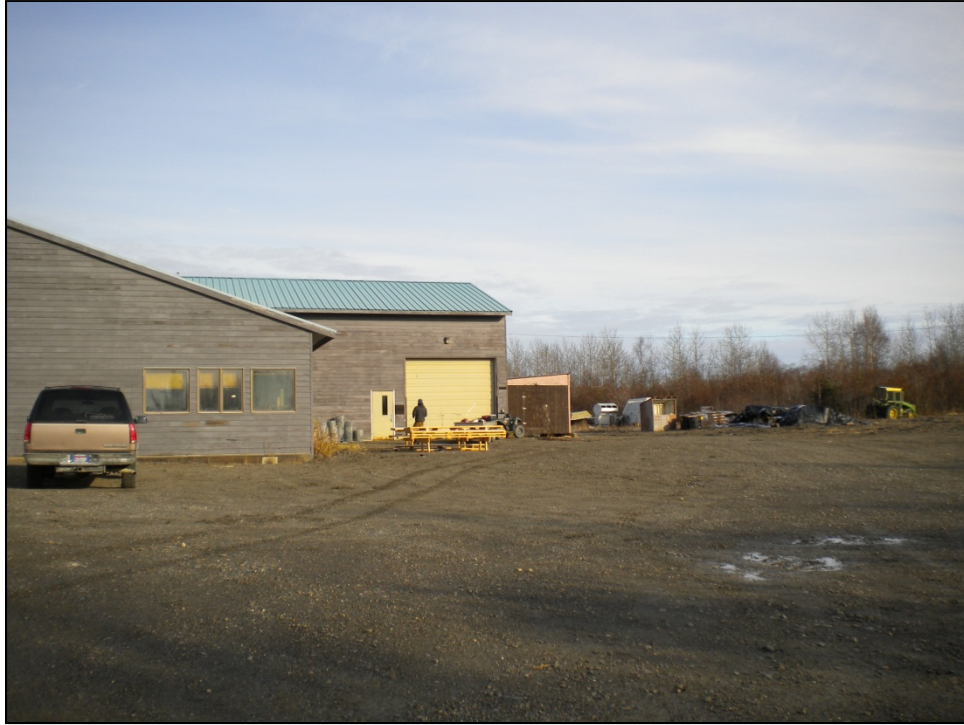
PHOTOGRAPH 1: LOOKING TOWARDS WOOD SHOP ENTRANCE FROM HIGH SCHOOL
