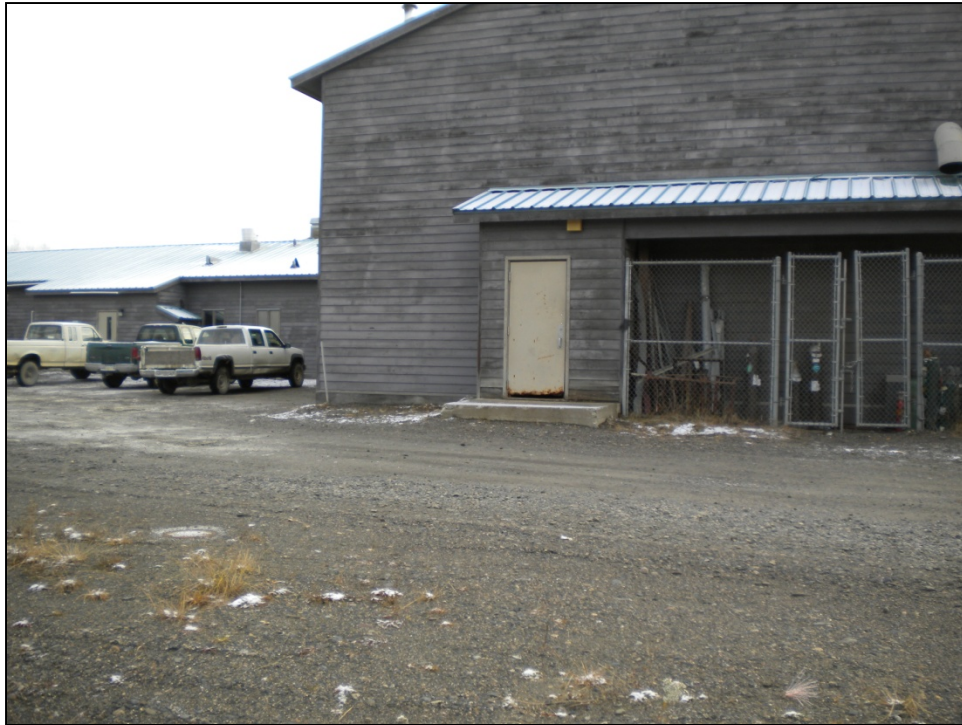
PHOTOGRAPH 9: TAKEN FROM MW-5 LOOKING TOWARDS BUILDING
