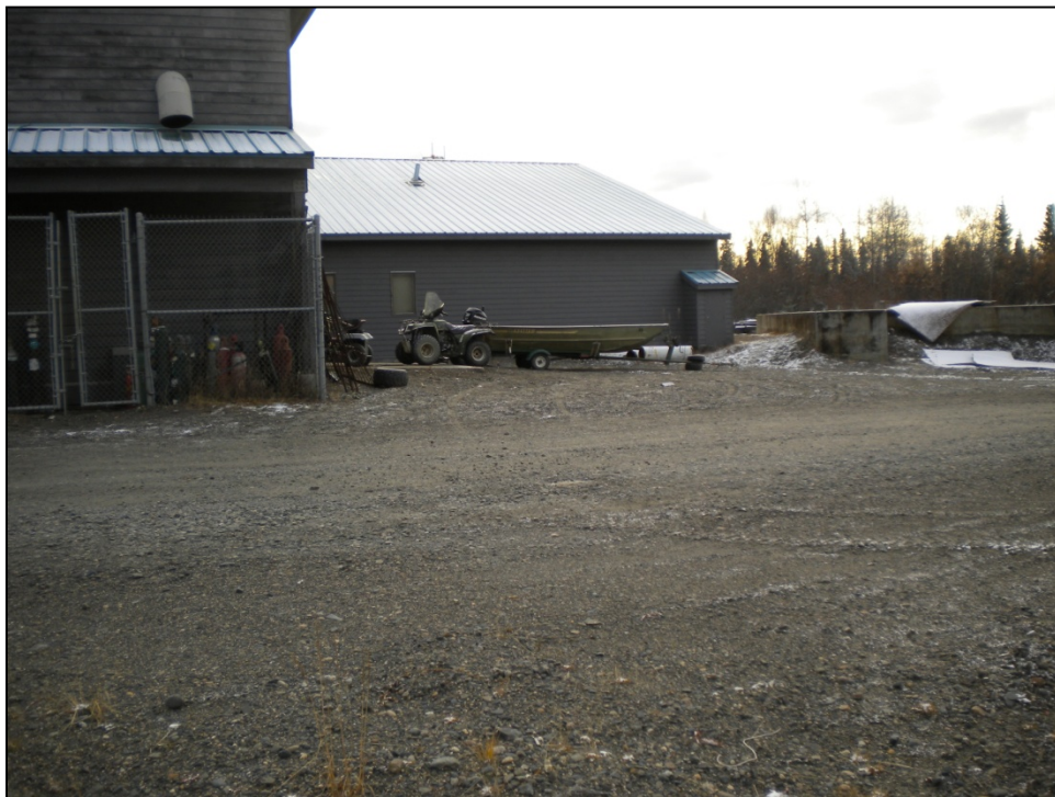
PHOTOGRAPH 10: TAKEN FROM MW-5 LOOKING TOWARDS S ANTENNA FOUNDATION
