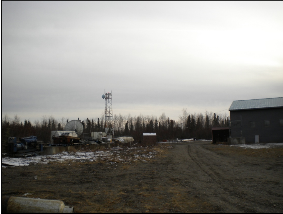
PHOTOGRAPH 3: TAKEN FROM MW-11 LOOKING TOWARDS E. ANTENNA FOUNDATION
