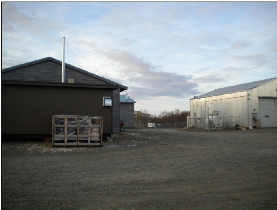
PHOTOGRAPH 6: TAKEN FROM BEHIND SYSTEM TRAILER LOOKING SOUTHWEST
