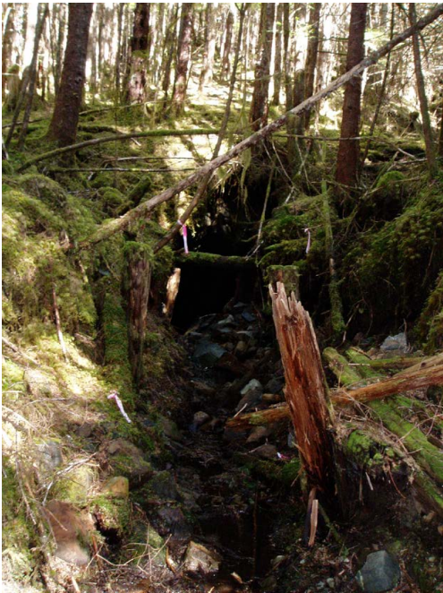
One of the main adits to the mine is shown in this May 2009 photo (above); the adit looked similar in the summer of 2011. An adit is a nearly horizontal passage from the surface to a mine. (DEC photo)
